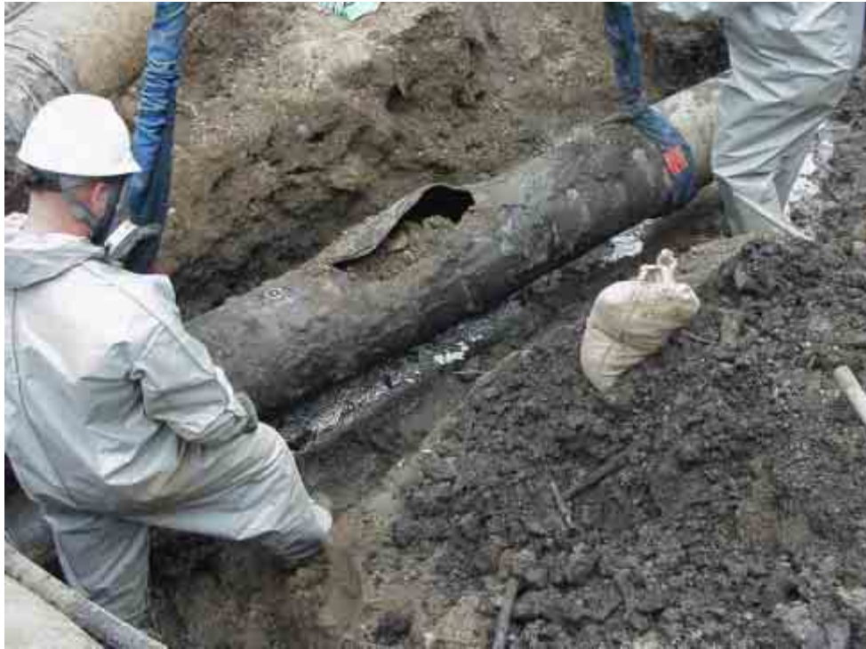
Figure 10. Removal of ruptured pipe section.
