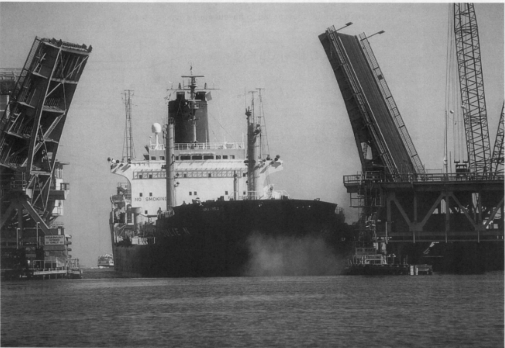
Figure 5—Accident site (photograph by Mr. Bill Jewel, Portland, Maine).
