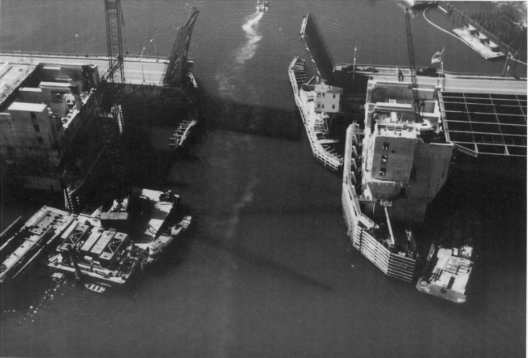
Figure 2—Aerial photograph of old and new bridges.
