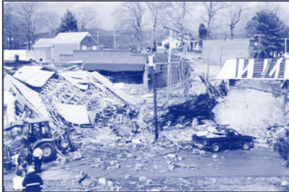
Bridgeport, Alabama natural gas explosion damage.
