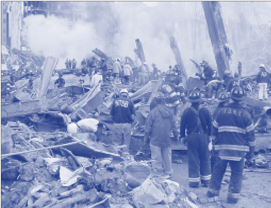
NTSB investigators on scene at the World Trade Center following the September 11, 2001 terrorist attack.
