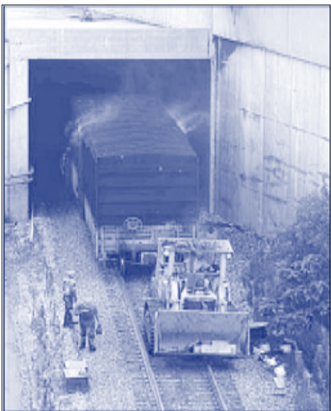
Rail cars being removed from tunnel.
