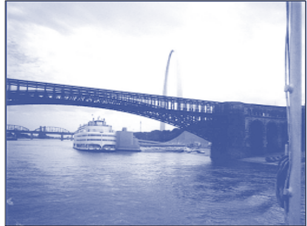
President Casino on the Admiral at its mooring complex below the Eads Bridge.
