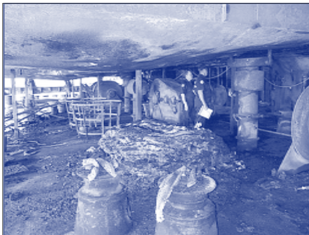
View of M/V Ecstasy 's fire damaged aft mooring deck.
