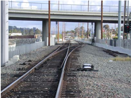
Figure 1: Accident location looking west.
