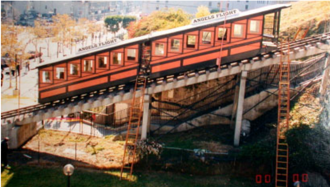
Figure 4. Ladders placed for the emergency evacuation. Walkway on the other side of the tracks can be seen below track level.
