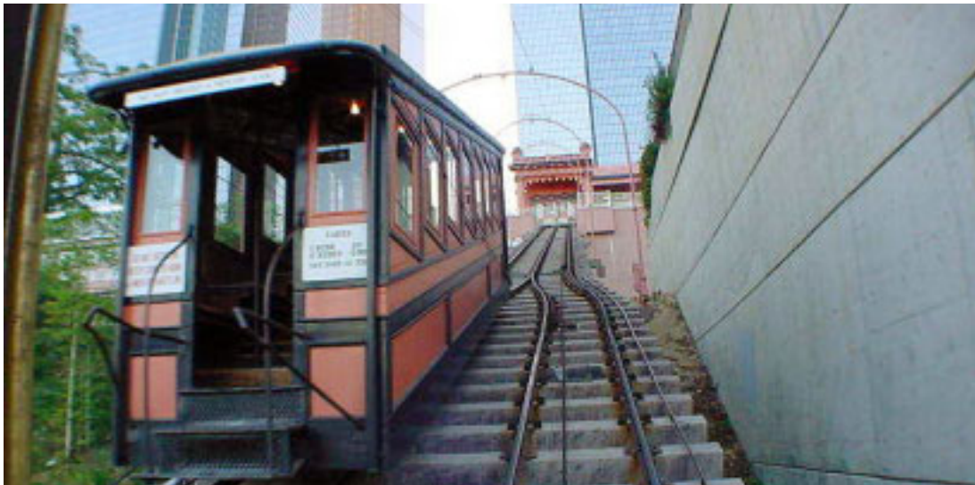
Figure 2. Angels Flight car at the passing siding with upper station in the background.
