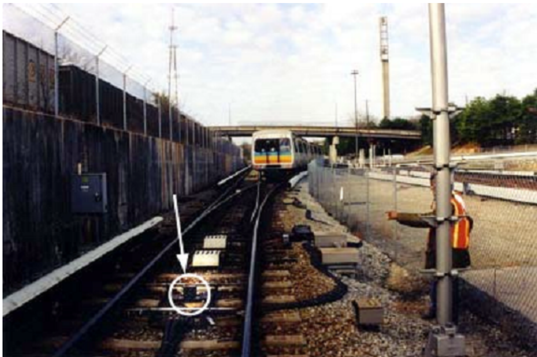
Figure 2. Train approaching the accident location from Avondale Station. The relay box that the technicians had opened is circled and indicated by the arrow.
