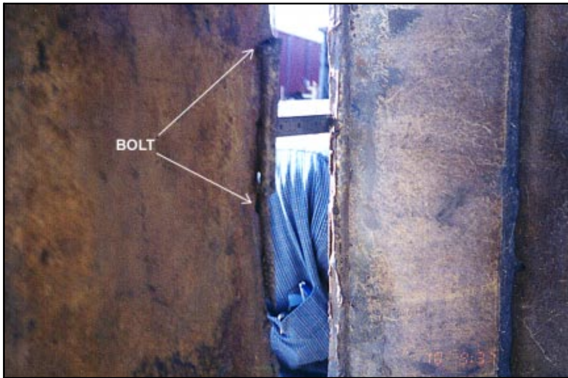
Figure 14. Bolt used to make improper repair to DTTX 72318
