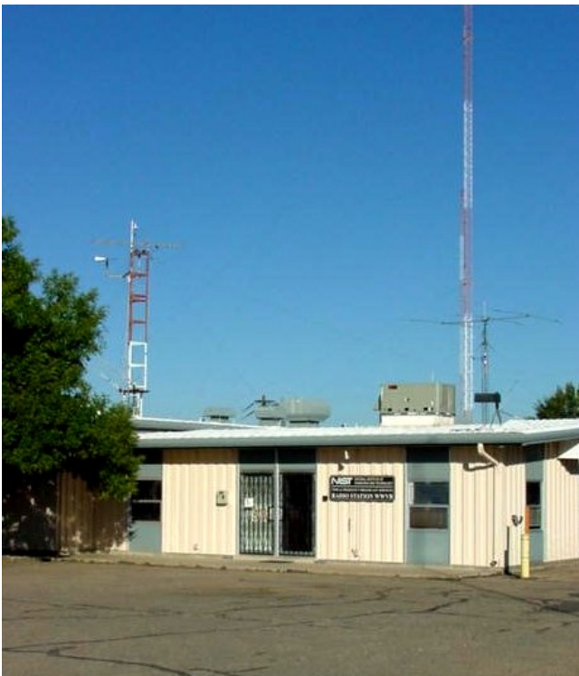
Figure 1.14. View of WWVB building.
