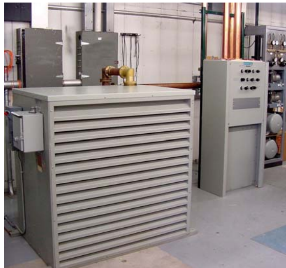
Figure 1.18. Dummy load and switch matrix..
