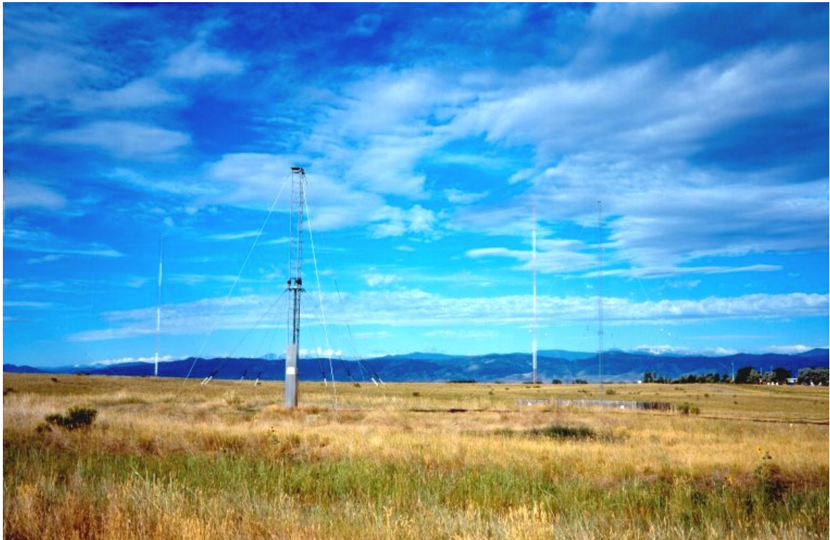
Figure 1.10. The 15 MHz antenna at WWV.
