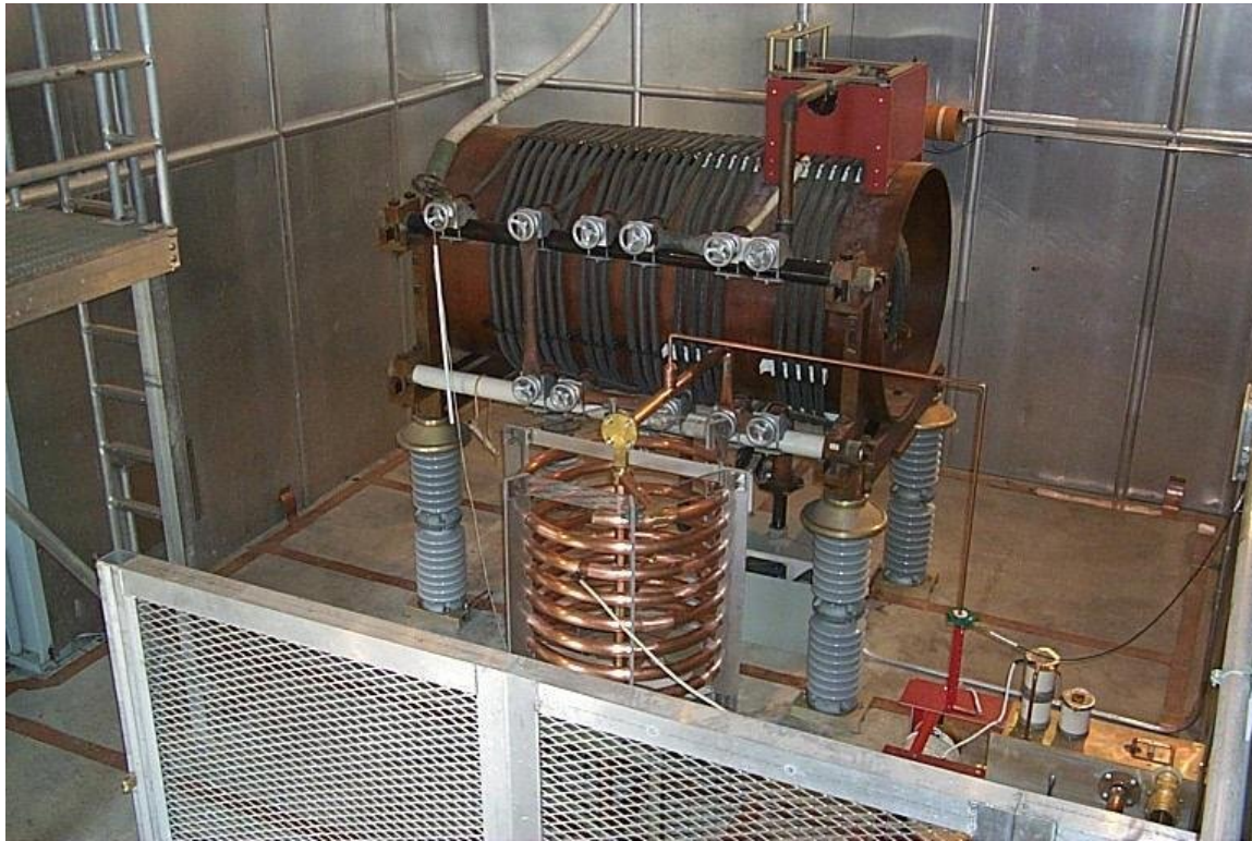
Figure 2.18. Interior view of helix house.
