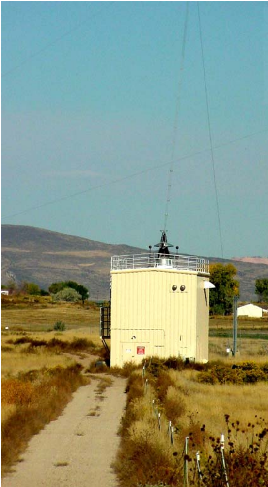
Figure 1.15. WWVB helix house.
