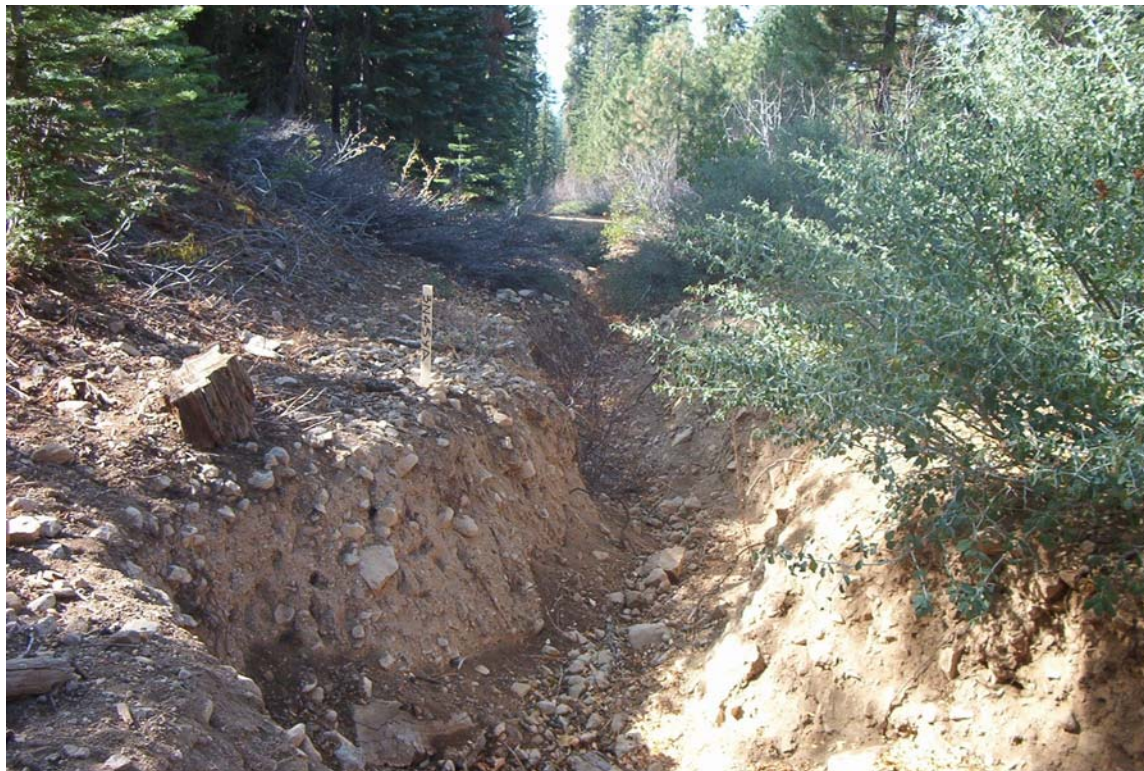
Photo 1, Gully erosion on Road 3N45YA
