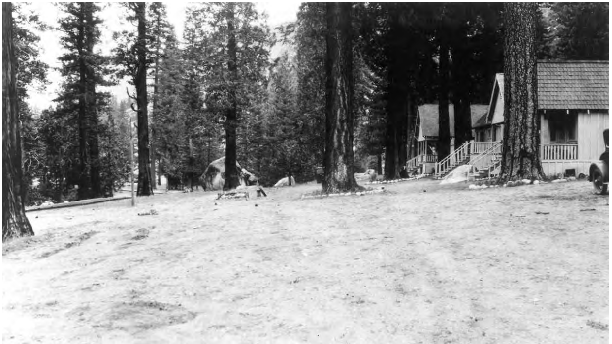
Baker Highway Maintenance Station, 1931. California State Archives Collection
