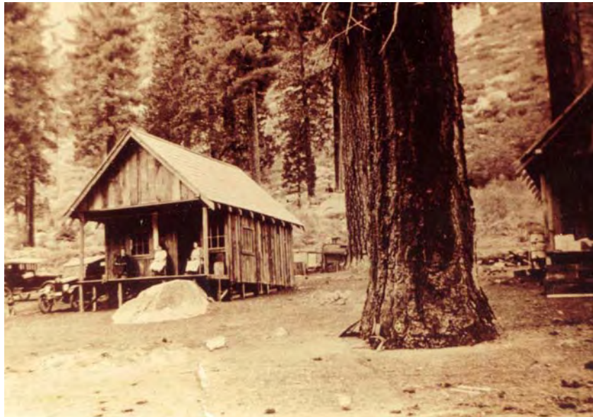
This photograph, reportedly taken in about 1920, shows the vertical board and batten siding, the ample, open front porch, the steeply-pitched front gabled roof, and the multi-light wooden windows that characterize the buildings constructed in the residential area for the Baker Highway Maintenance Station, completed in about 1931 or '32. Typically, the cottages for state highway maintenance stations were roofed with composition asphalt shingles; the roofs at Baker were wood shingles.
