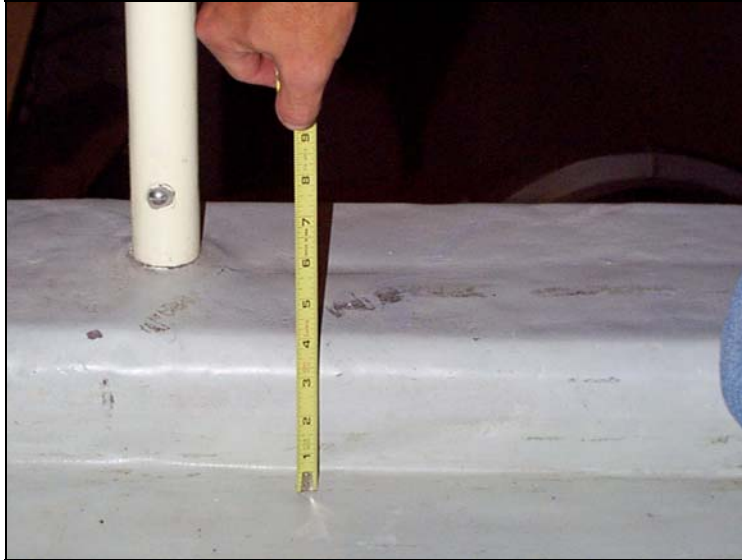
Figure 2. Typical Concrete Curb
