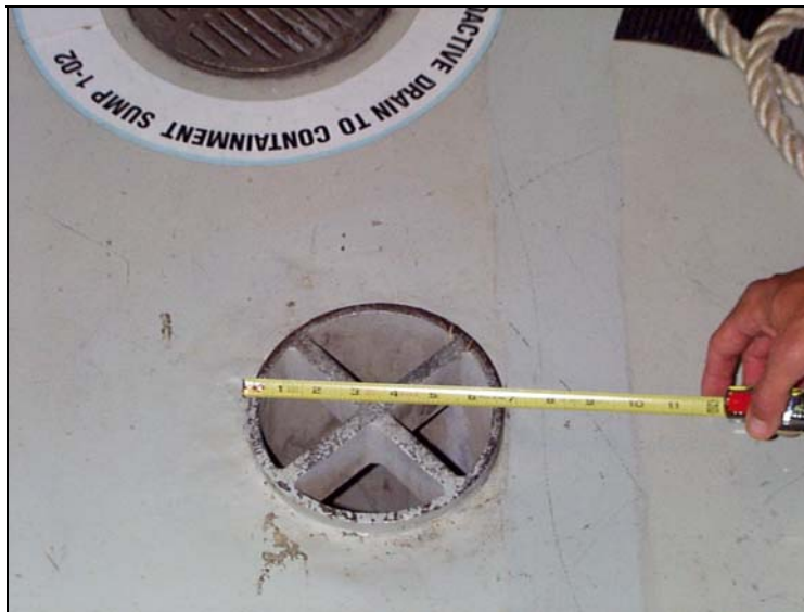
Figure 1. Typical Floor Drain
