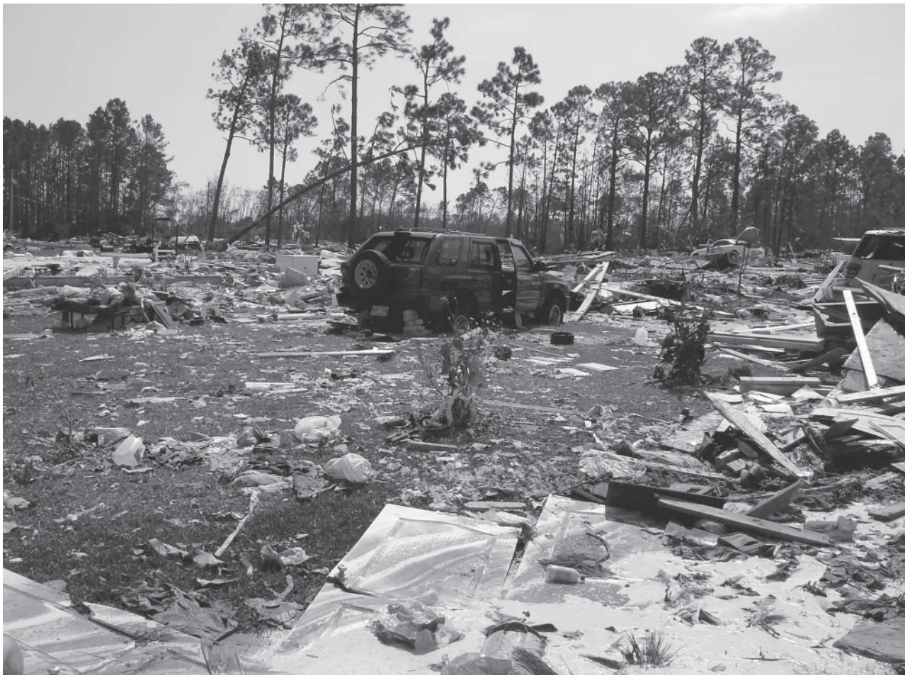
Hurricane's destruction: Outside of D'iberville and St. Martin, MS. These were single family houses. (Photo courtesy of LCDR Hall-Robinson.)
