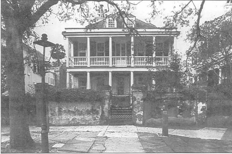
FIGURE B.3 The first building code in South Carolina was a document developed by and for Charleston in 1907. (Photo: The Charleston Area Convention and Visitors Bureau)
