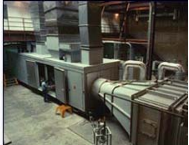
Figure 2-4. Rolls-Royce Allison 501-K Turbine Power Package
