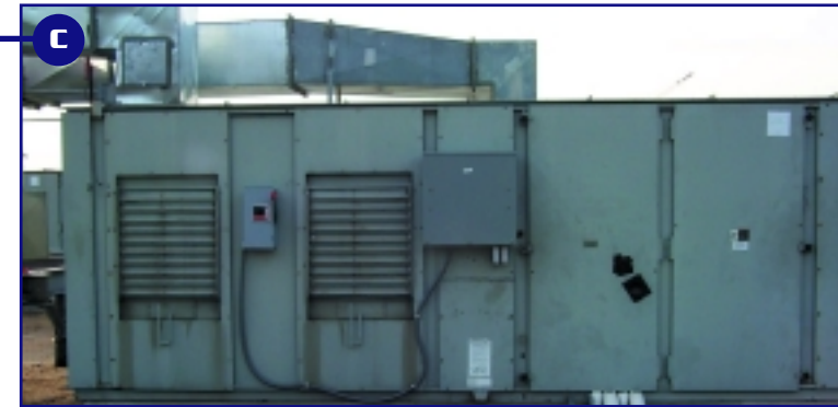
Rooftop air conditioning unit (RTU)
