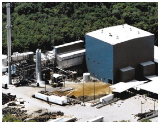
Figure 5-3. The Exeter Energy Facility burns 100 percent tire-derived fuel
