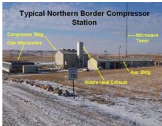
Figure 23. Compressor Station Overview Pictures
