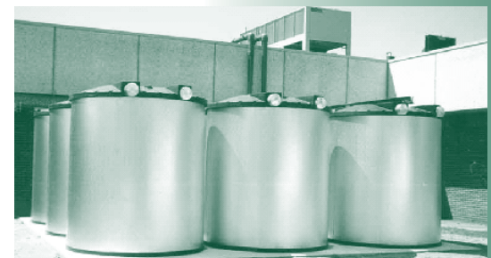
Conventional Thermal Storage Tanks
