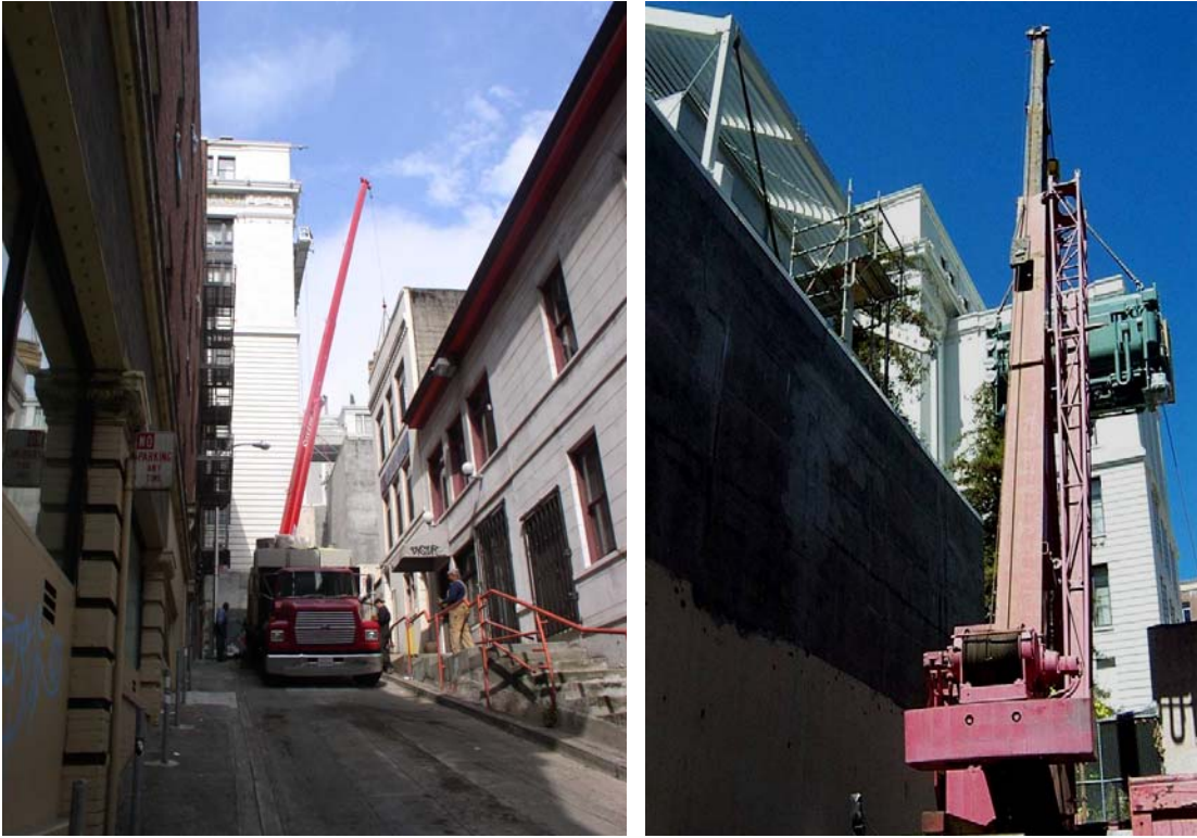
Figure 11 Hoisting the Chiller
