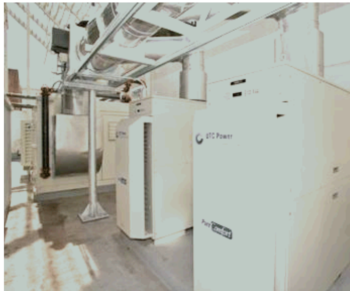
Figure 8 CHP System Layout on Ritz-Carlton Rooftop
