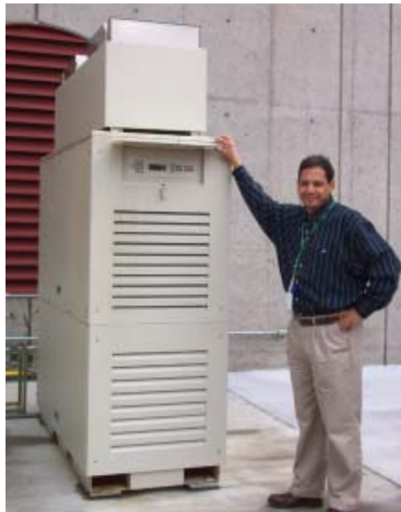
Capstone microturbine - 60 KW
