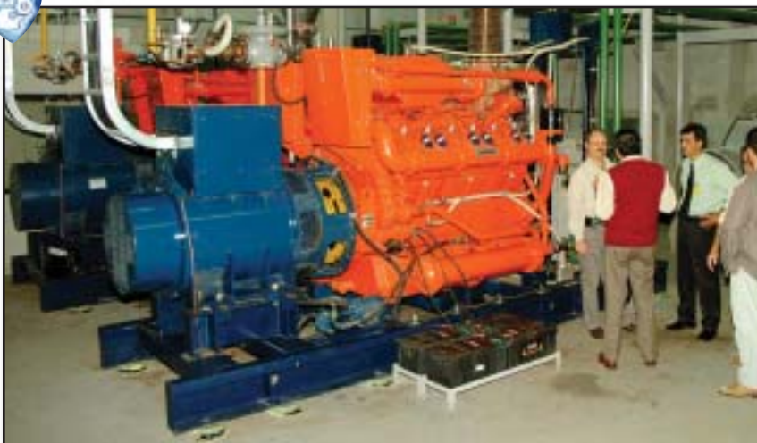
Each engine manufacturer is using a specific engine platform for applying their ARES development work and technologies. Waukesha Engine is using its venerable VGF Series. Pictured is a VGF P48GLD, rated 800 kW.
