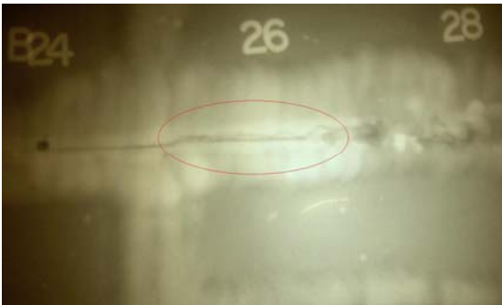
No. 6- Portion of radiograph of weld at CH-18 C3, view 20-34. Dark line (circled) is a crack in the weld.
