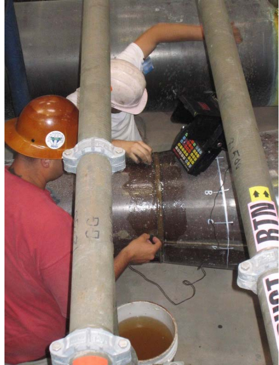
No. 7- Shear-wave ultrasonic testing. The weld is coated with gel couplant and ultrasonic transducers on angled blocks are moved over it. Image on instrument is interpreted by technicians to indicate presence or absence of defects.
