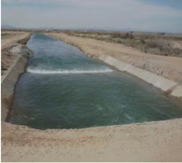
Broad Crested Weir in Earthen Canal
