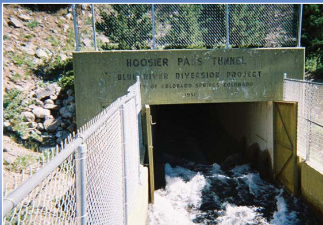
Hoosier Pass Tunnel
