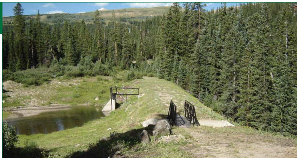
West Hoosier Creek Diversion
