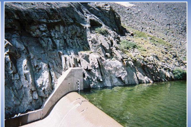
Upper Blue Reservoir Spillway
