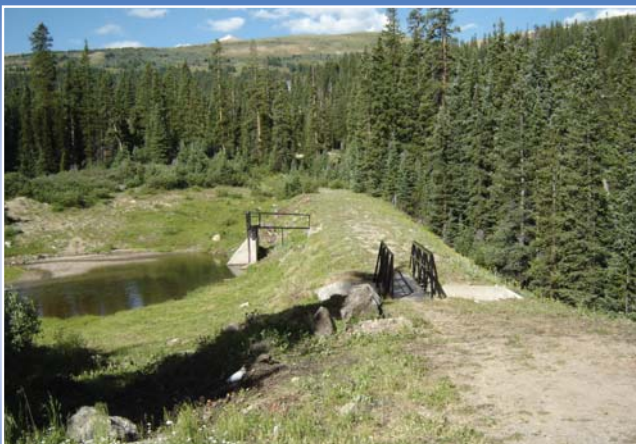
West Hoosier Creek Diversion
