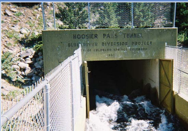
Hoosier Pass Tunnel
