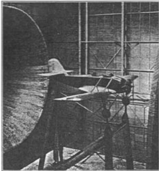
FIGURE 1.—The McDonnell airplane with large fillet in full-scale wind tunnel.
