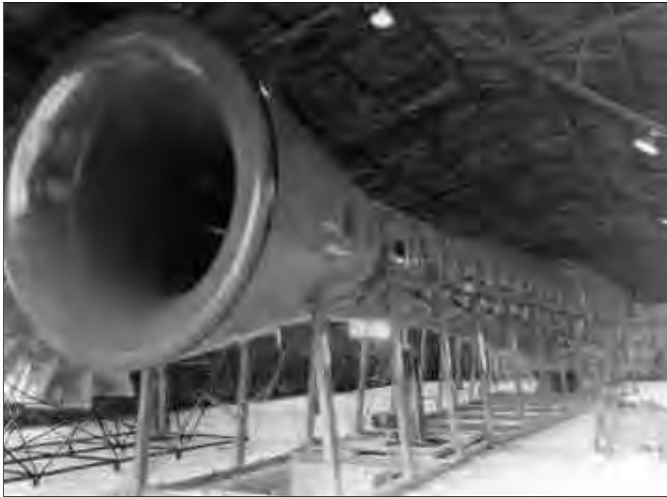
The U.S. Army's first-ever wind tunnel, built at McCook Field in Ohio in 1918, could reach extremely high speeds for its day. It had a twenty-four-blade fan that spanned five feet in diameter, which could push the airspeed (within its small fourteen-inch diameter closed-throat test area) to a little over 450 miles per hour. The tunnel is now on display in the Air Force Museum in Dayton. SI Negative No. A-1855
