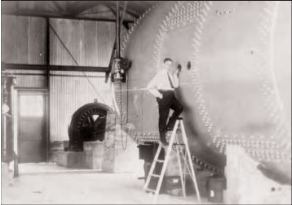
Dr. Max M. Munk, the Variable Density Tunnel's creator, inspecting the machine not long after its installation. One peered into the machine through two small portals on the side. NASA Image #EL-1999-00258 (LaRC)
