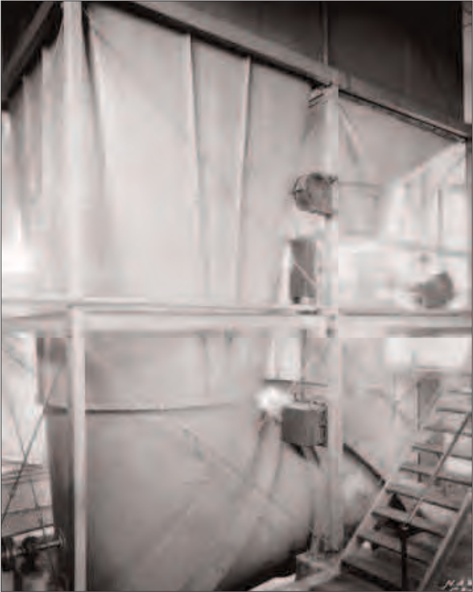
Housed in the same building as the seven- by ten-foot AWT, Langley researchers used the five-foot Vertical Wind Tunnel mainly for spin tests. An engineer kneels on a platform next to the test chamber. In the foreground is the device's (closed) return passage. Like the AWT, the tunnel had an open throat. The vertical tunnel stood thirty-one feet tall and was twenty feet long and ten feet wide. It was not ready for operation until early 1931. NASA Image #EL-1999-00410 (LaRC)
