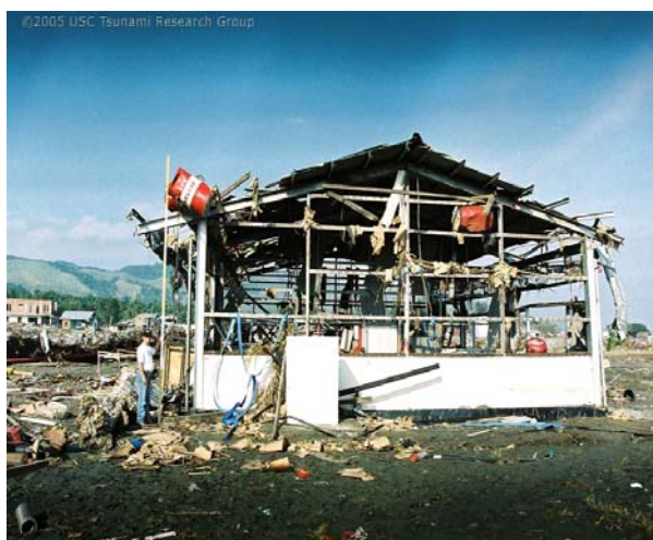
Earthquake engineering researchers from the University of Southern California recorded details of the destruction from the December 2004 South Asian earthquake, including the height of debris left by the subsequent tsunami. The researcher holds a 5-meter-high rod against a house in Panteraja, Sumatra. Credit: © Jose C. Borrero, University of Southern California Tsunami Research Group, http://www.usc.edu/dept/tsunamis
