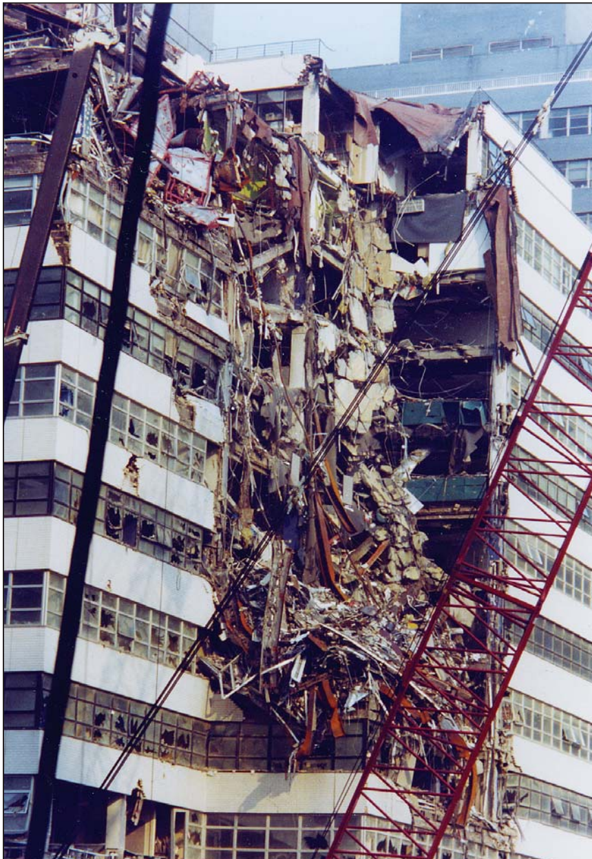
Figure 7-13 30 West Broadway – south façade, 6th floor to roof, looking northeast.
