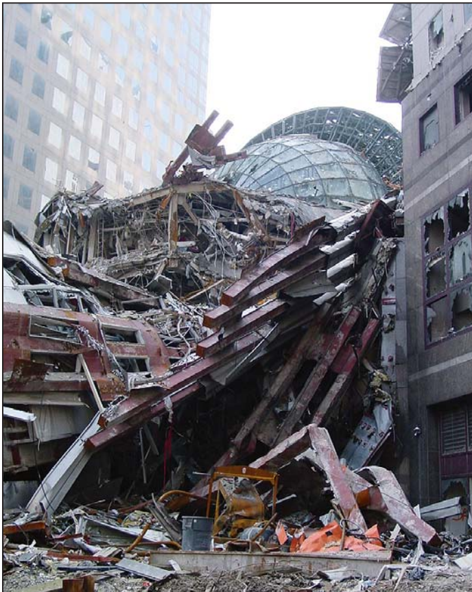
Figure 7-4 View of Winter Garden damage from West Street, with WTC 1 debris leaning against WFC 3.
