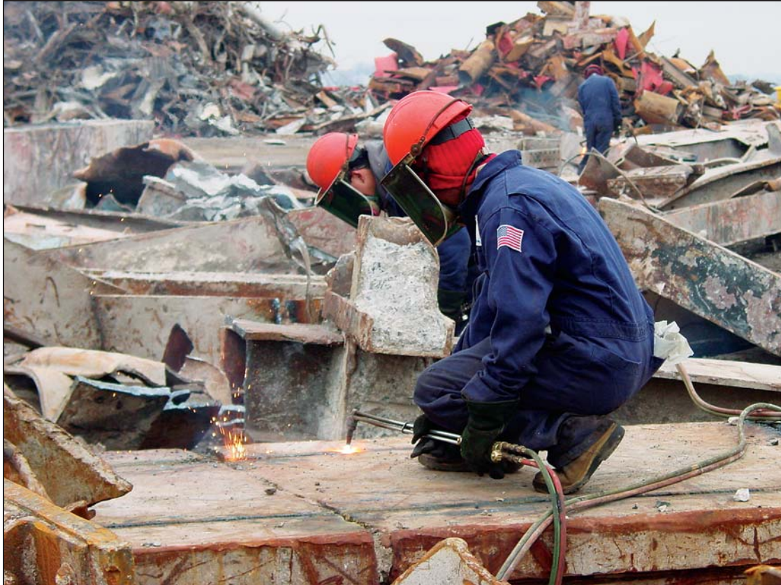
Figure D-2 Torch cutting of very large pieces into more manageable pieces of a few tons each.
