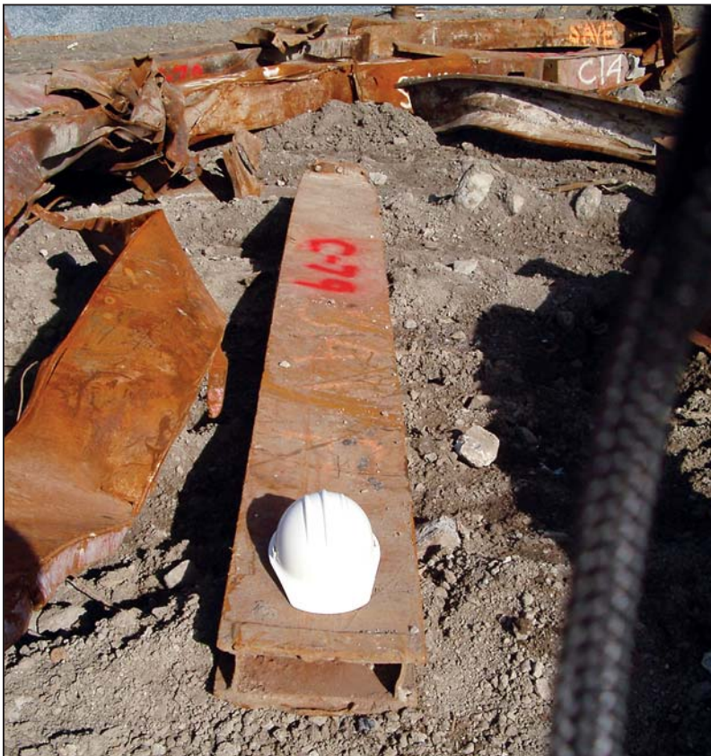
Figure D-13 WTC 1 or WTC 2 core column (C-74).
