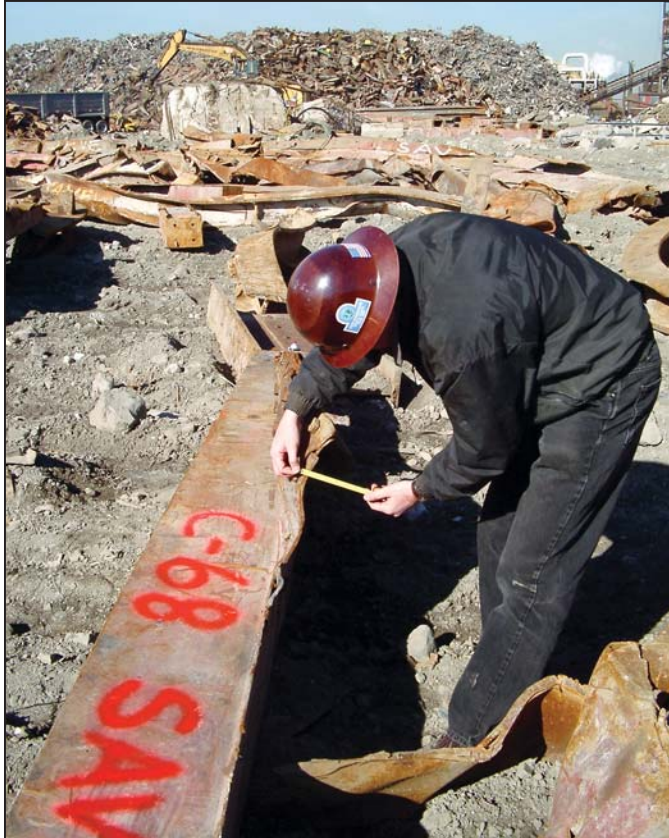
Figure D-8 Engineer measuring spandrel plate thickness ( t_s ).
