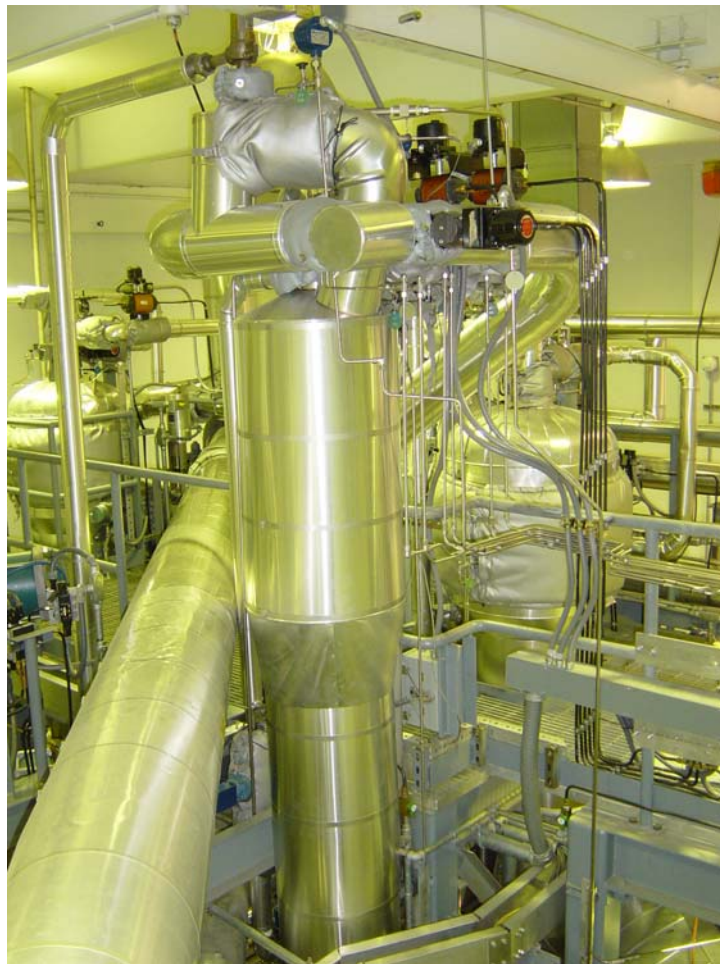
Figure 3.5. Photograph of Pressurizer in the APEX Facility
