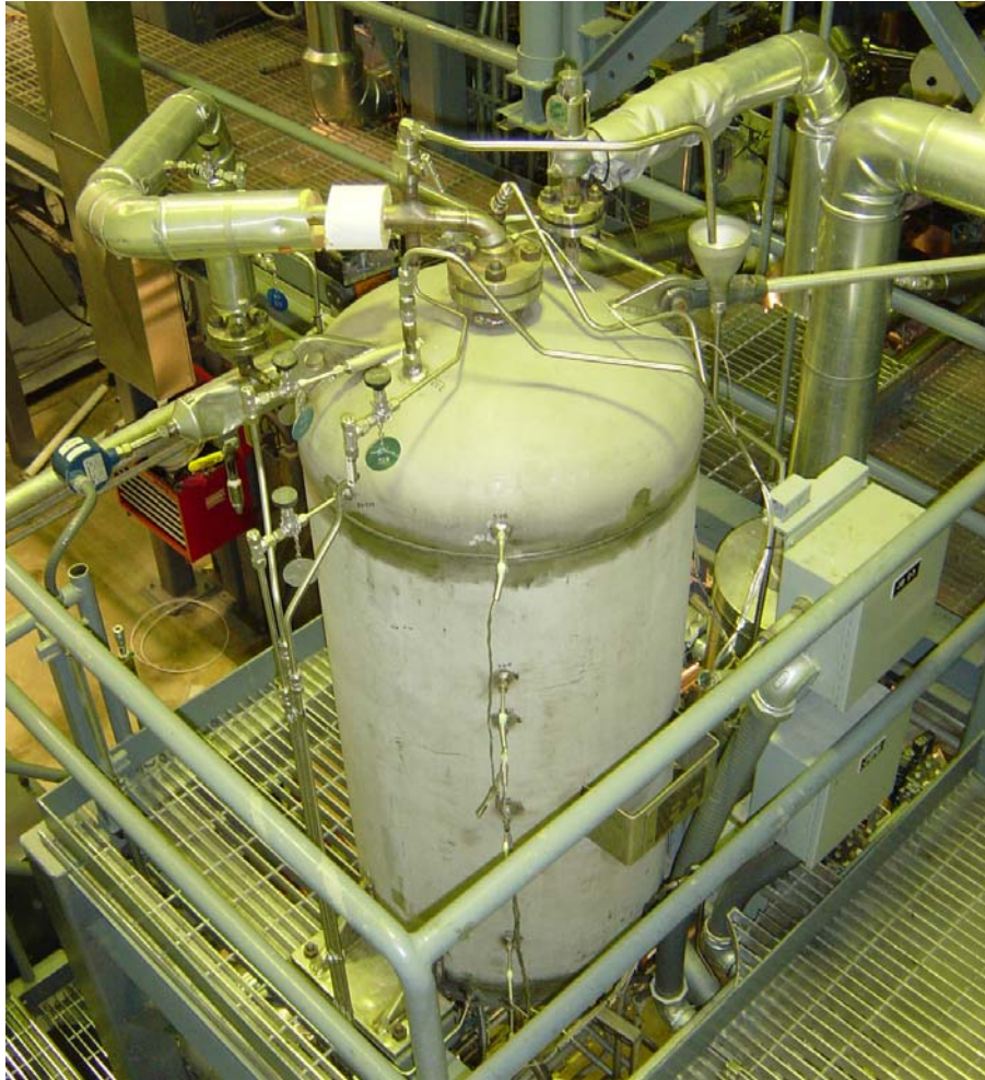
Figure 3.16. Photograph of a Core Makeup Tank
