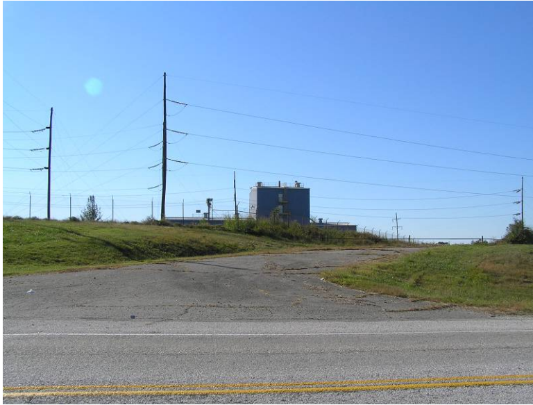
Looking west at Proposed Disposal Cell Area from Highway 10
