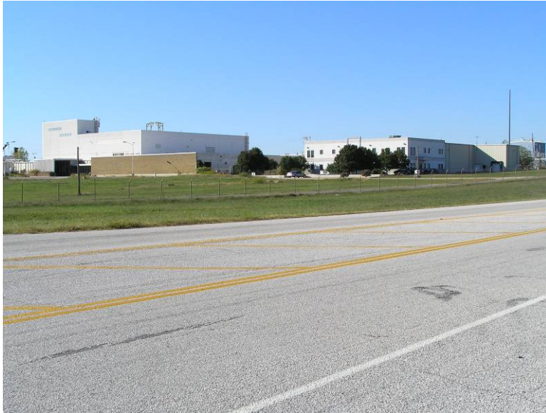
Southeast side of SFC Process Area from Highway 10
