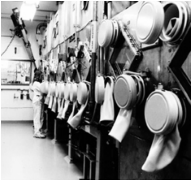
Glovebox Workstations in Building 371
