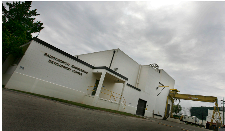
DOE Building 7920 of the Radiochemical Engineering Development Center (REDC)
