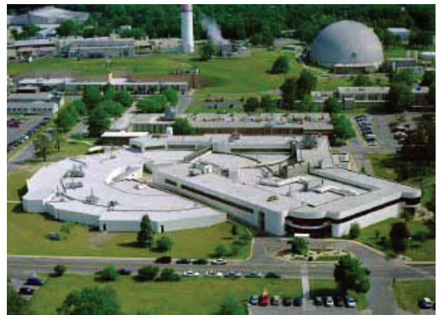
Aerial view of NSLS
