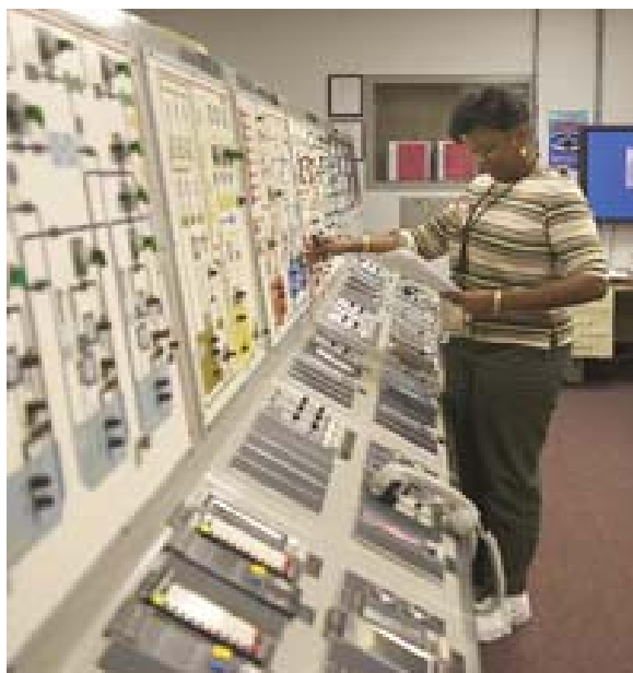
HB-Line Control Room
