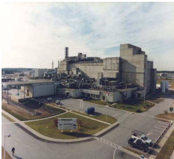
Aerial View of SRS
