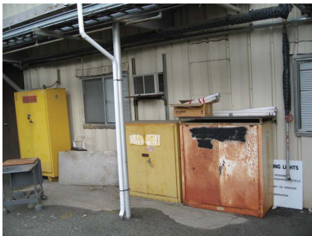
An Unlabeled Waste Accumulation Area
