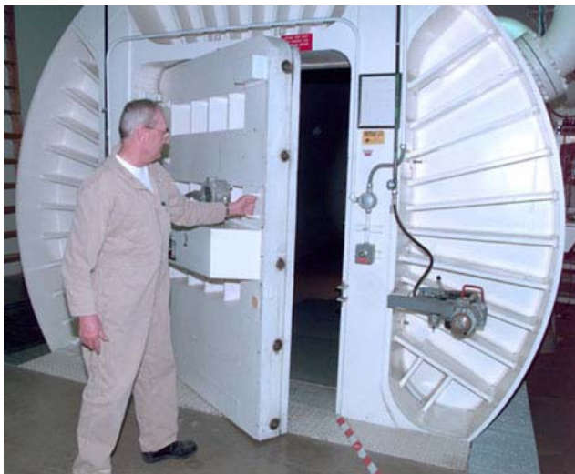
Isolation Door at the Pantex Plant
