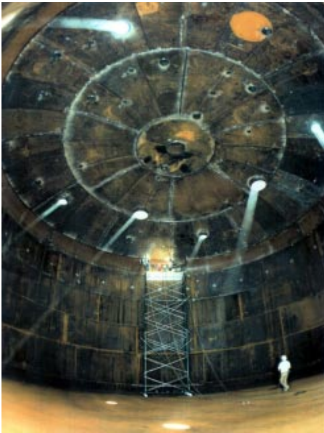
Inside a Waste Tank
