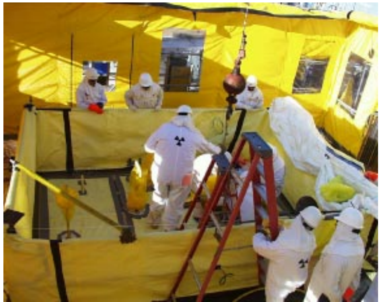
Workers in Pit, January 2000
