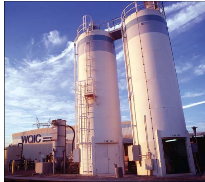
Water Quality Improvement Center, Yuma, AZ
