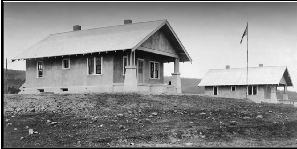
Figure 1.86 Strawberry Valley Project, Utah. Watchmen's cottages at East Portal of Strawberry Tunnel, 1914. Frame Bungalow houses with stuccoed exterior walls and metal shingle roofs.
