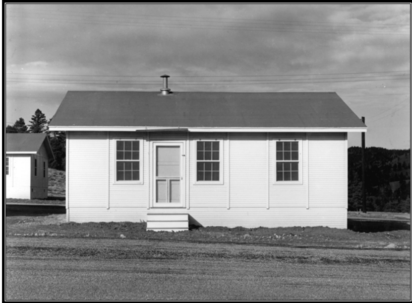
Figure 4-21. Missouri River Basin Project, Canyon Ferry Unit. Temporary prefabricated house is similar to ones installed at Davis Dam camp. Photo taken November 4, 1948.
