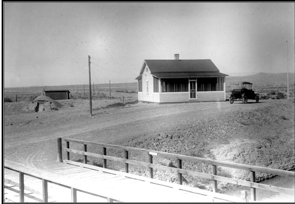
Figure 1.46 Grand Valley Project, Colorado. Ditchrider's quarters, Little Salt Wash, 1919. Built in 1916, the house has screened porches off the front and rear elevations.
