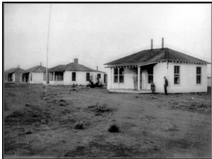
Figure 1.25 Huntley Project, Montana. View of permanent buildings at headquarters camp, September 7, 1905. Simple hipped roof cottages with covered porches were a common Reclamation building type.
