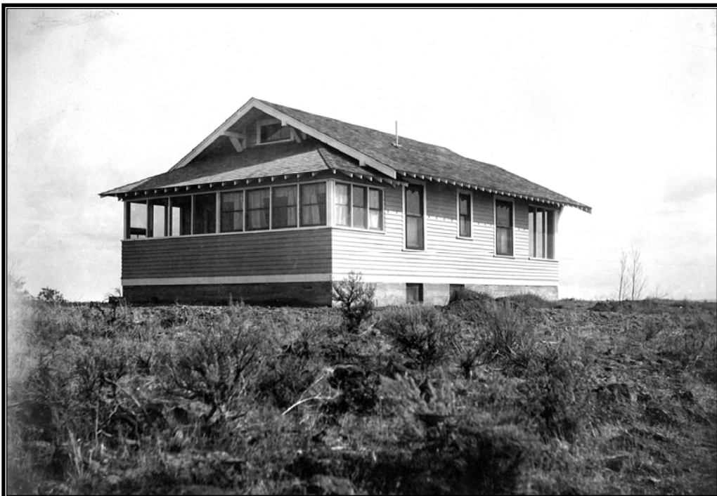
Figure 1.89 Rear view of 1914 cottage at Minidoka Dam camp showing screened sleeping porch. Each cottage contained a living room, dining room, kitchen, bathroom, and one bedroom.
