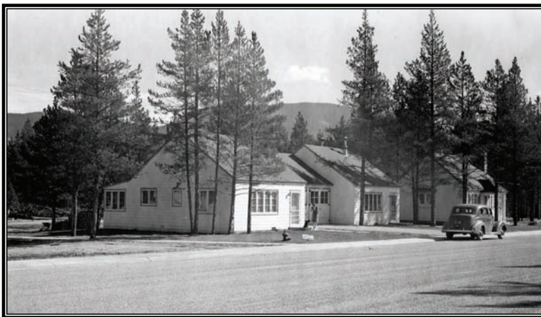
Figure 3.45 Duplexes at Shadow Mountain camp in October 1940. Each unit within a duplex contained a living room, kitchen, bedroom, bath, large glassed porch at the rear, and a garage.
