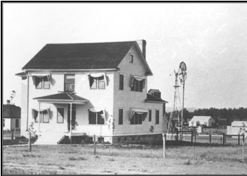
Figure 1.57 Milk River Project. Headquarters building in Malta, Montana. Just visible to the left side is a two-story concrete vault original to the building. Deviations in construction from the original blueprints were numerous and included Doric columns rather than turned porch posts, a reference to the Colonial Revival style.
