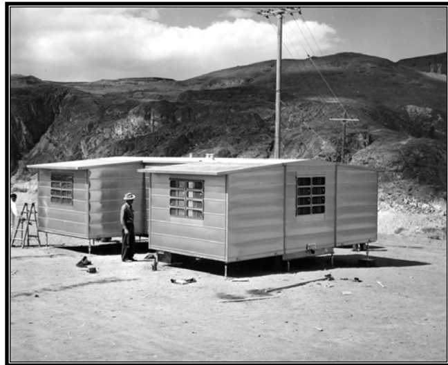
Figure 4.4 Transa-Home after being unfolded and opened into a five-room house. Photo taken April 25, 1950.
