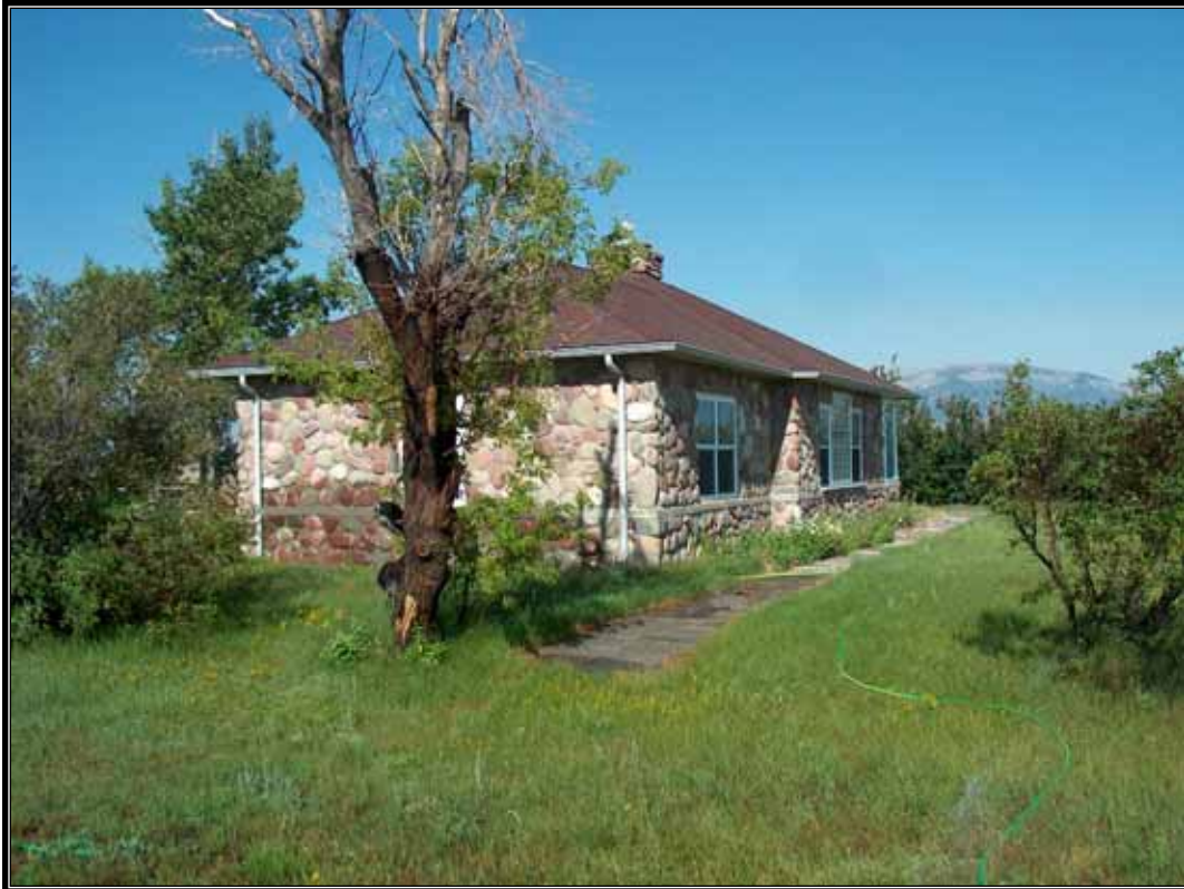
Figure 3.78 Sun River Project. Recent view of cobblestone CCC buildings at Pishkun Reservoir. (Source: Montana Area Office, Bureau of Reclamation)
