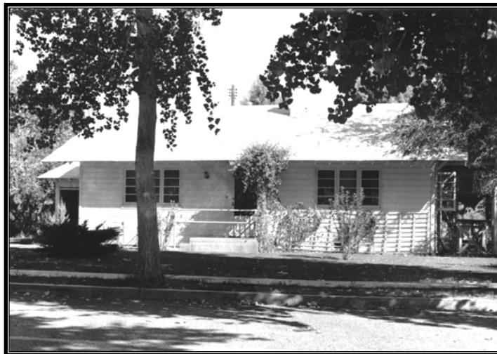
Figure 3.58 Parker Dam camp, building number 25. Undated photograph.
