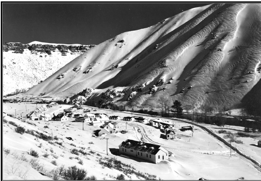
Figure 3.53 Anderson Ranch Dam camp in January 1943. Large building in foreground is a dormitory. Permanent buildings are to the left of the street in front of the dormitory.
