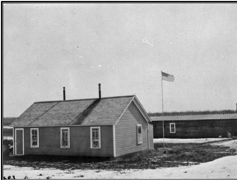
Figure 1.40 Lower Yellowstone Project. Newly completed office building at La Mesa camp in September 1905, prior to extension added the same year. In the drafting room, 2-inch by 8-inch floor joists were used rather than 2-inch by 6-inch joists to lessen vibration for men engaged in drafting.
