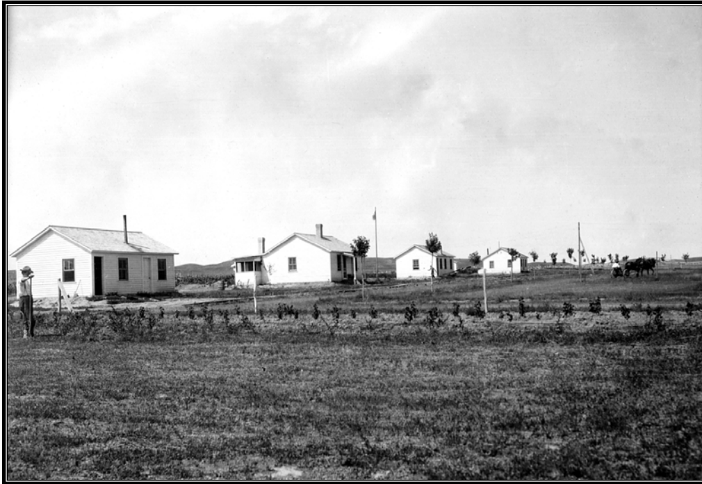
Figure 1.23 Lower Yellowstone Project. Ridgelawn camp, circa 1910. Recently planted trees can be seen towards foreground. Temporary office building is second from right with flag in front.
