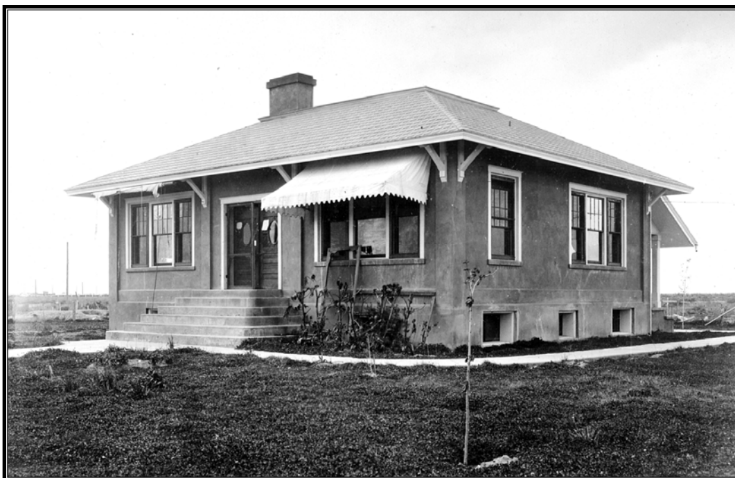
Figure 1.63 Minidoka Project. Reclamation office in Rupert, Idaho, 1909. Craftsman style influences are clearly seen in the kneebraces under the extended eaves and the multi-paned over single-paned windows.
