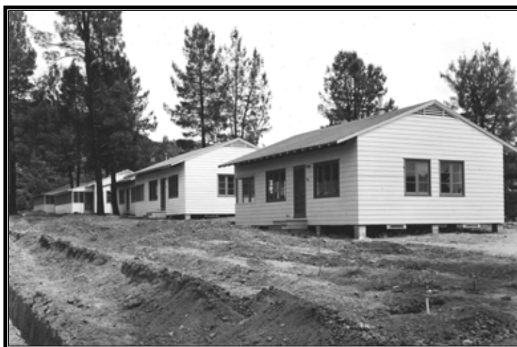
Figure 3.47 Four-room residence at Toyon built according to standard Denver drawing number 40-D-2412 for a type 5, four-room residence. Photo taken June 1938. (Source: Northern California Area Office, Bureau of Reclamation)
