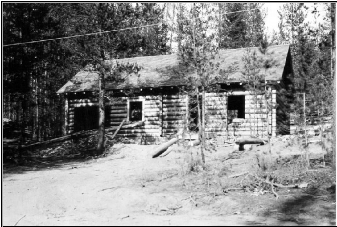
Figure 3.66 View of cabin number 2 at Deadwood Dam under construction in September 1929.
