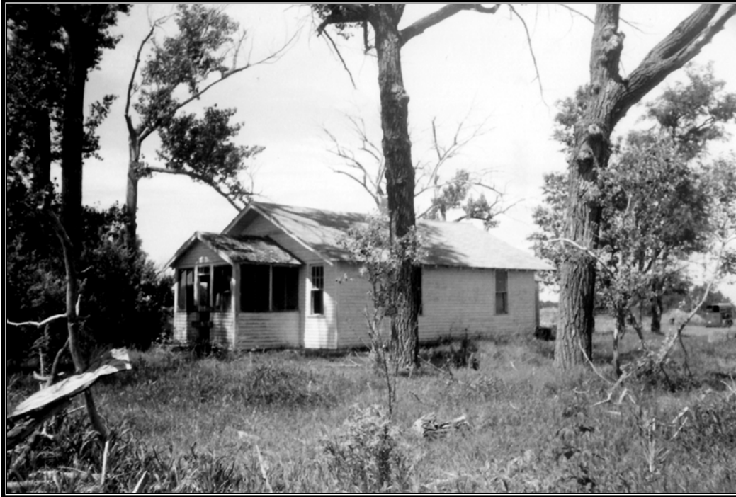
Figure 1.39 Belle Fourche Project. Ditchrider's house is listed in the National Register of Historic Places. Although abandoned, the house retains historic integrity. Reclamation realizes the high interpretive potential of the site. (Source: Jim Kangas, Bureau of Reclamation)
