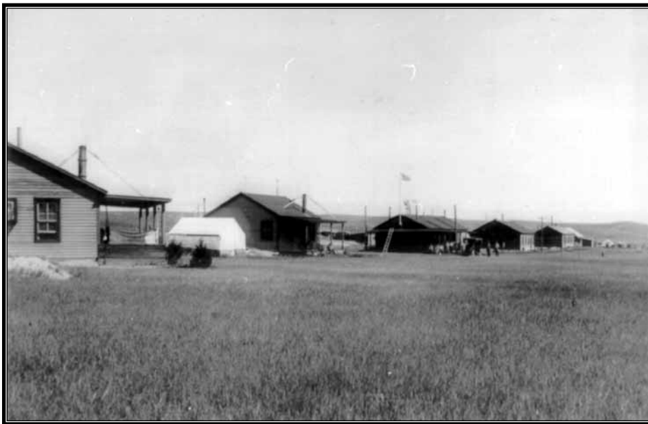
Figure 1.21 Lower Yellowstone Project. Temporary buildings at La Mesa headquarters camp, 1910.
