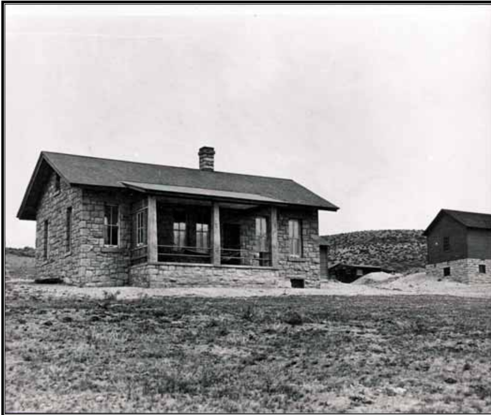
Figure 1.38 North Platte Project, Wyoming. Pathfinder dam tender's house built of local stone, 1909.
