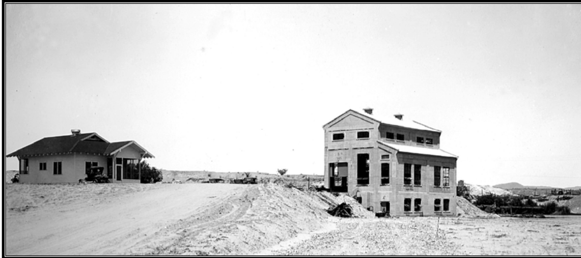
Figure 2.15 Yuma Project. New Siphon Drop Powerplant operator's house shown in 1926 photo. Nearly identical to the 1918 standard four-room cottage plan, this house featured a large roof ventilator rather than chimneys.
