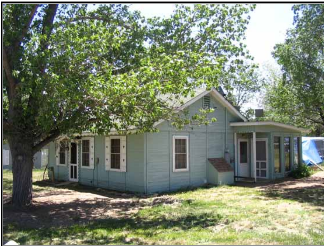
Figure 4.14 Colorado-Big Thompson Project. Example of Reclamation prefabricated house still exists at Estes Park. See figure 4.21 for similar type constructed at Canyon Ferry. Photo taken June 2007. (Source: Christine Pfaff, Bureau of Reclamation)
