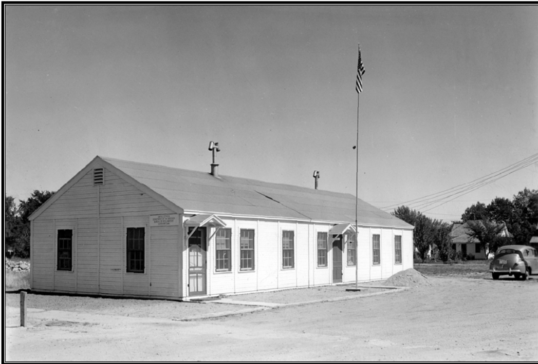
Figure 4.18 Missouri River Basin Project, Narrows Unit. Office in Fort Morgan. Photo taken September 21, 1948.
