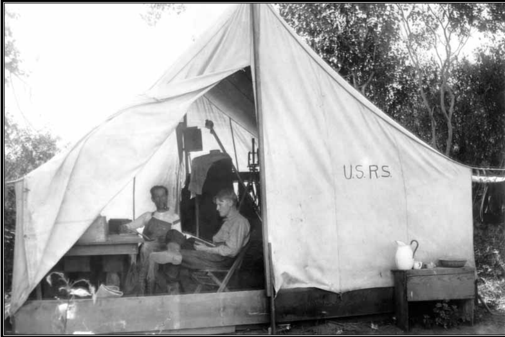
Figure 1.4 Yakima Project, Washington. Reclamation headquarters at Sunnyside Canal, September 23, 1907.
