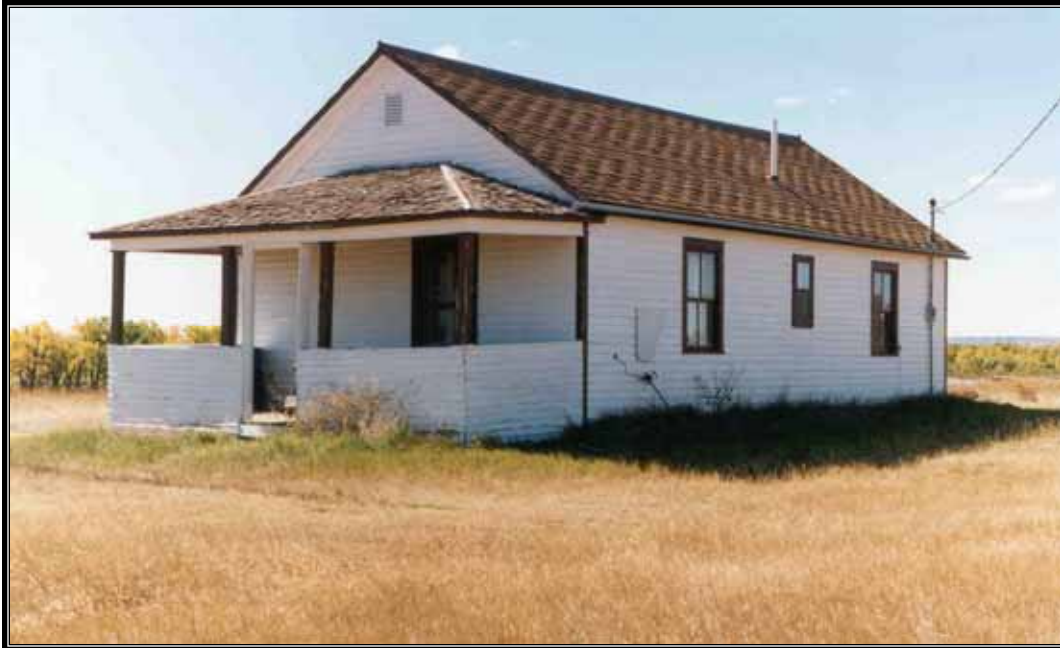
Figure 1.30 Lower Yellowstone Project. Headworks camp, office building converted to dam tender's house, 1997. The basic form remains unaltered, but the entrance and porch have been moved to the gable end. (Source: Mary McCormick, Renewable Technologies, Inc.)
