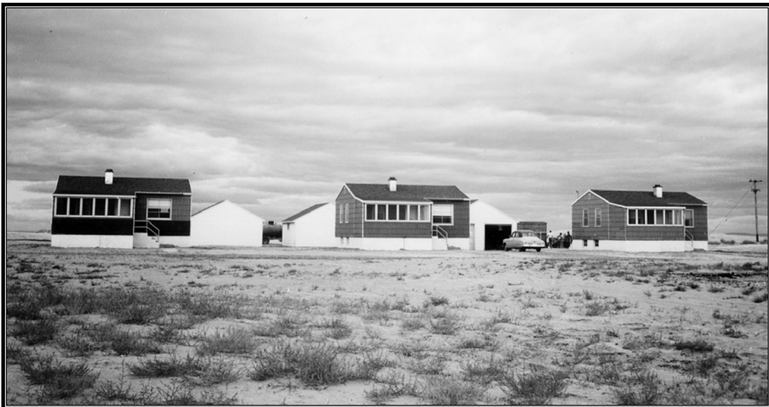
Figure 4.8 Columbia Basin Project. Completed houses at Ringold Pumping Plant sit on raised concrete foundations. Photo taken September 23, 1953.
