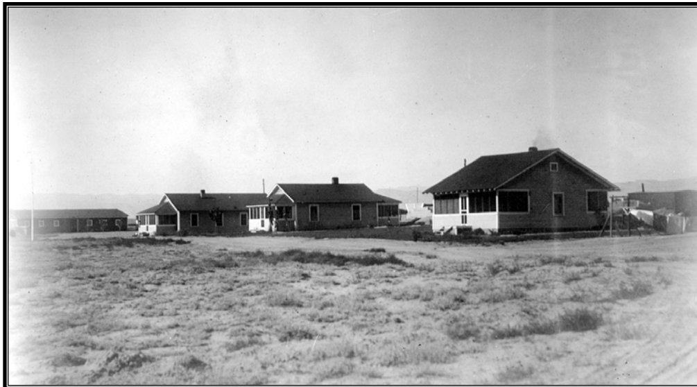
Figure 1.37 Grand Valley Project, Colorado. Permanent buildings at Maintenance Camp 7, 1919.
