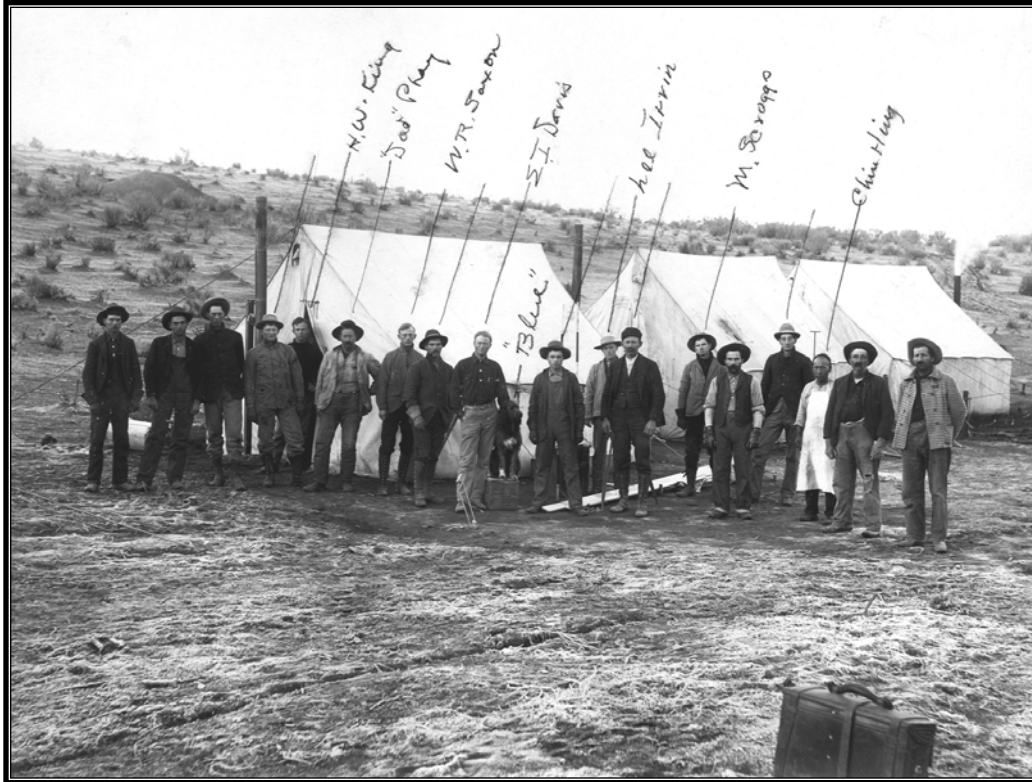
Figure 1.2 Umatilla Project, Oregon. Cold Springs Dam survey camp, October 27, 1905. At the center of the photograph is "Blue" the dog.
