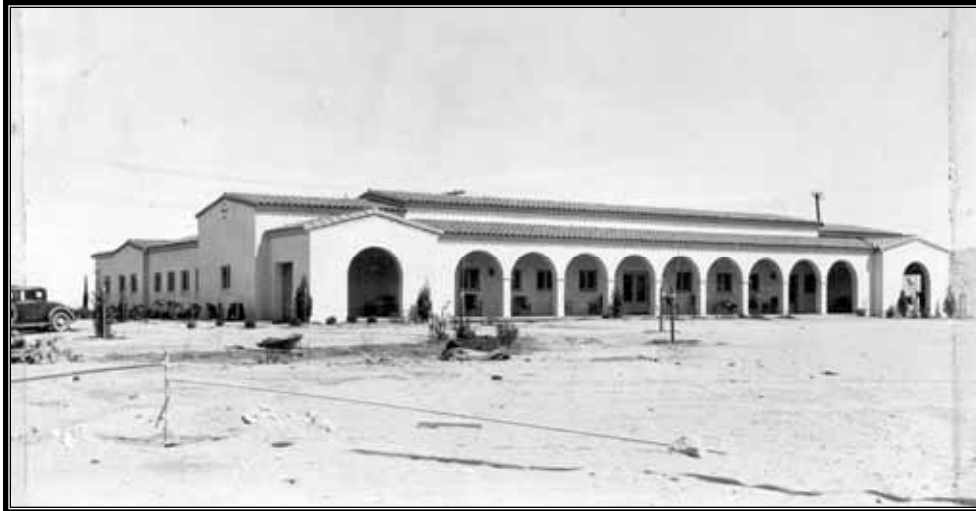
Figure 3.9 Boulder City dormitory in April 1932. Landscaping being installed adds the finishing touches. (Source: Reclamation photograph database)
