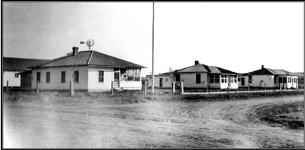
Figure 1.26 Huntley Project. Relocated camp buildings in Ballantine, circa 1920. Left to right: partial view of storehouse, office, project manager's cottage, chief clerk's cottage.
