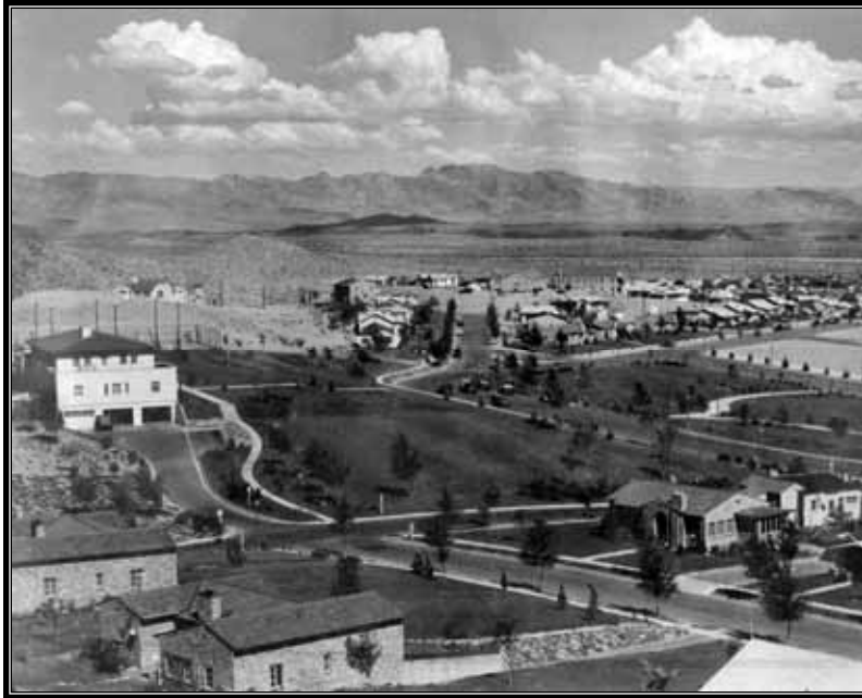
Figure 3.20 View from Water Tank Hill showing houses along Denver Street in the foreground. At center left is the administration building overlooking the park. Photo taken July 27, 1934.
