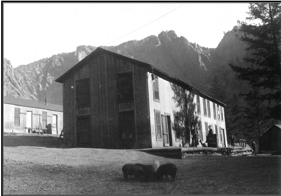
Figure 1.78 Uncompahgre Project. Office at River Portal, Colorado, 1907. Siding appears to be sheet metal or building paper. Pigs feed in the foreground.
