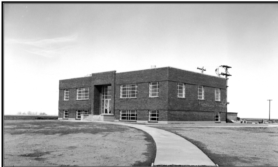
Figure 4.12 Columbia Basin Project. New division office building in Othello, Washington. Photo taken March 30, 1951.
