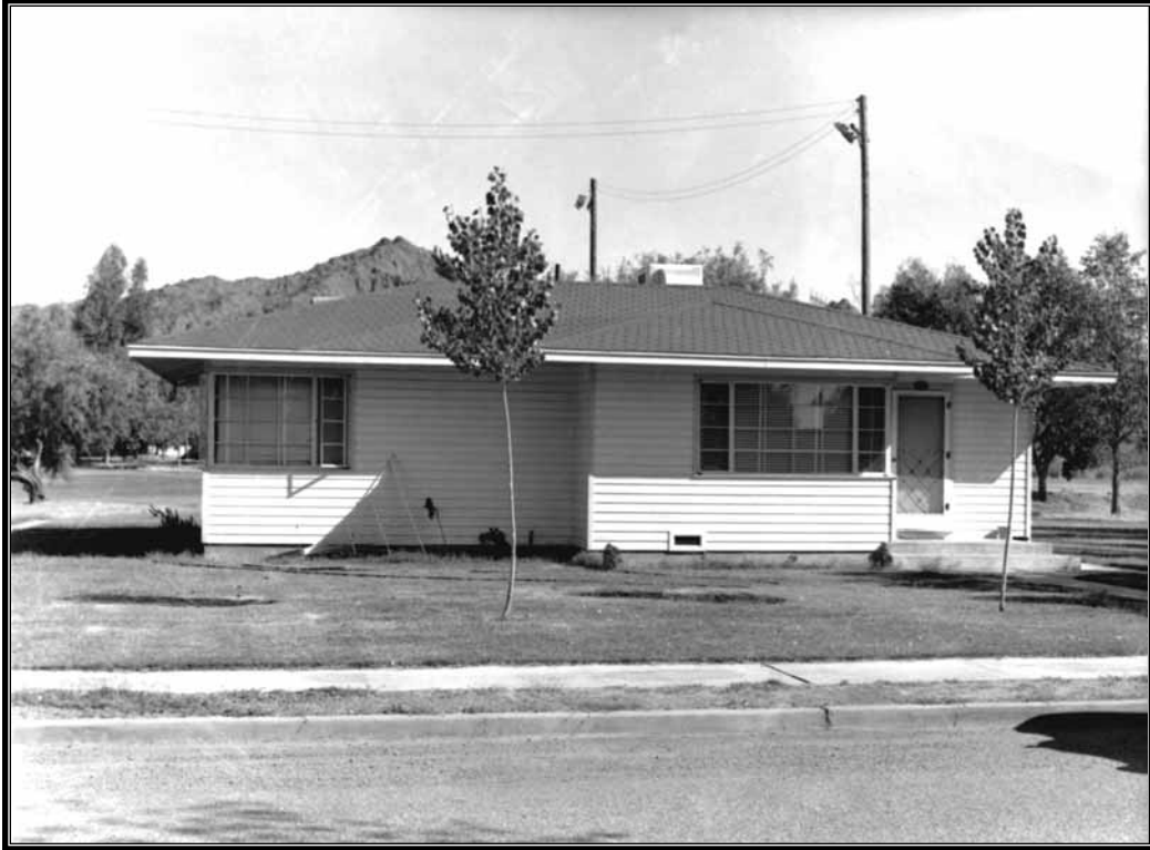
Figure 4.28 Parker Dam Camp. Permanent residence. Note broad overhanging eaves for sun protection. Photo date unknown.
