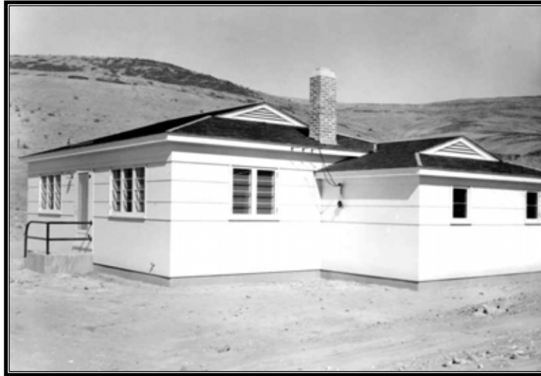
Figure 3.56 This house on the Roza Division of the Yakima Project was built in 1941, also using Denver standard drawing number 40-D-3191. Photo taken shortly after completion.
