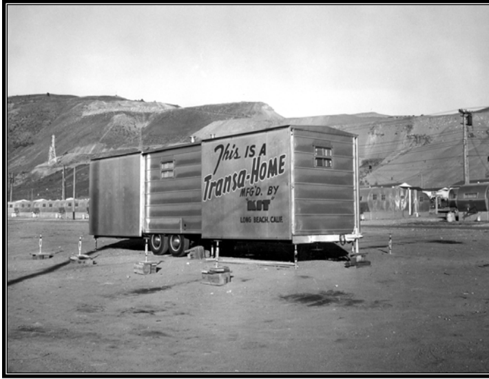
Figure 4.3 Portable Transa-Home as it appeared upon arrival at Coulee Dam in 1950.
