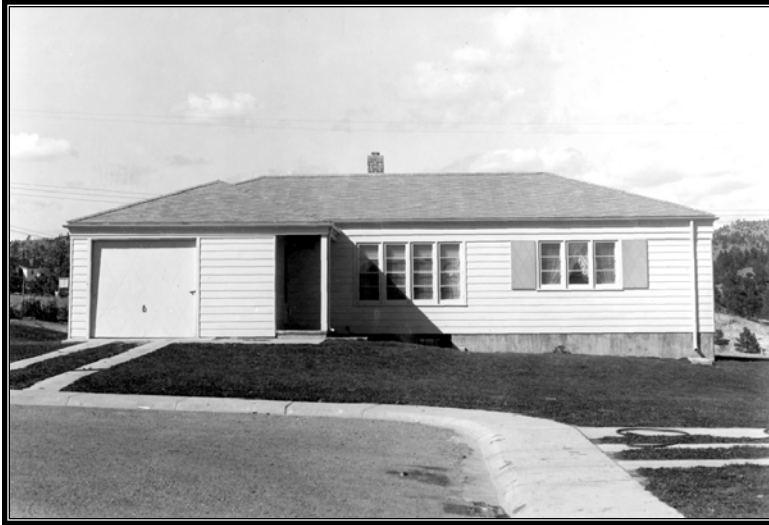
Figure 4.25 Canyon Ferry Unit. Six-room permanent house. Photo taken September 12, 1949.
