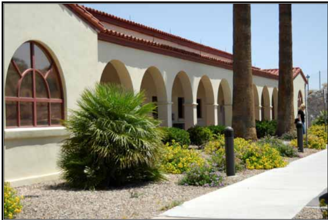
Figure 3.10 Boulder City dormitory now serves as office space and is called the Annex. (Source: Andy Pernick, Bureau of Reclamation)
