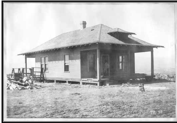
Figure 1.34. Yakima Project. Irrigation manager's house at Tieton Unit headquarters nearing completion, July 1910. Projecting eaves and exposed rafter ends show transition to Bungalow form. (Source: Upper Columbia Area Office, Bureau of Reclamation)
