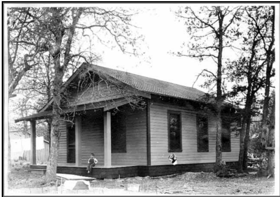
Figure 1.47 Yakima Project. Patrol house number 5 at South Fork Crossing, Tieton Unit, May 1911. The use of front-gabled roofs was far less common than side gables on Reclamation buildings. Shingles along building foundation contrast with the horizontal siding. (Source: Upper Columbia Area Office, Bureau of Reclamation)
