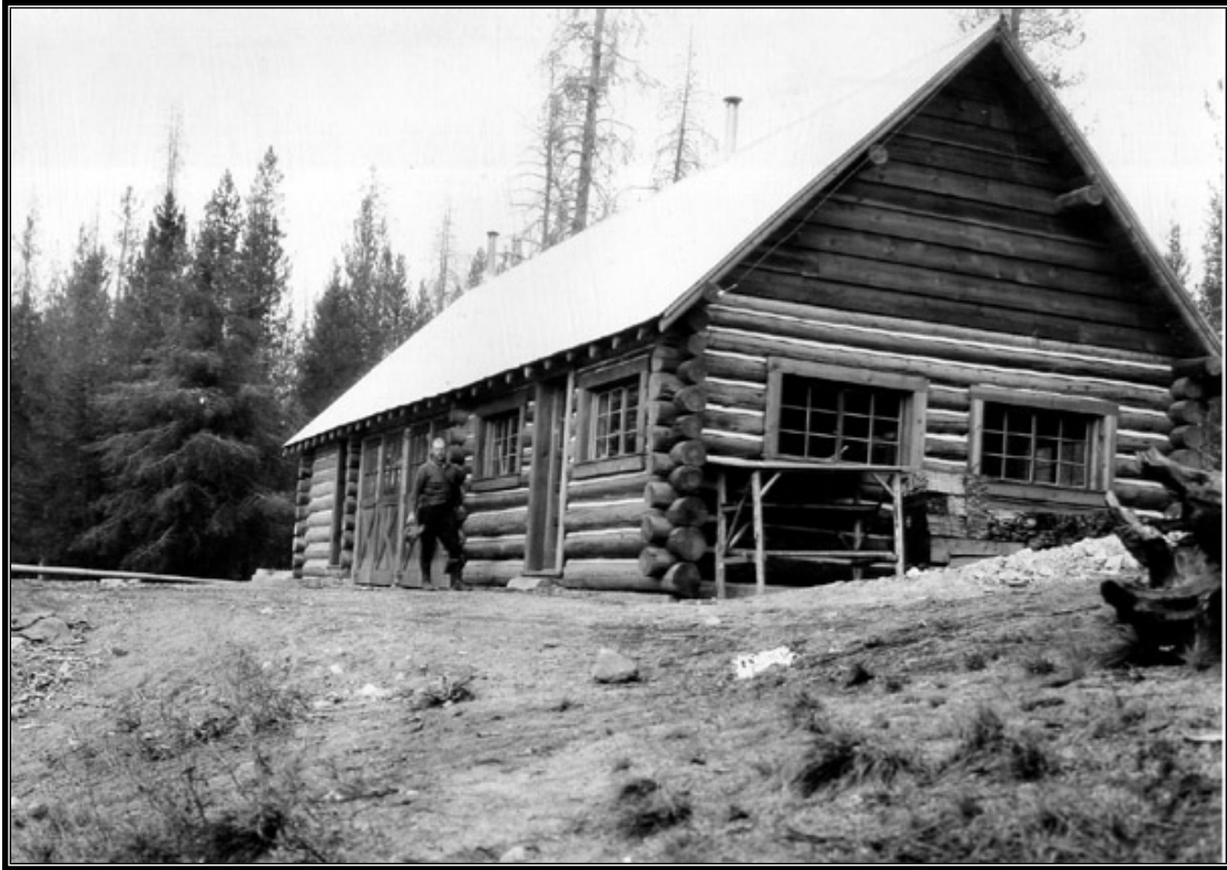
Figure 3.65 Boise Project. Deadwood Dam office during construction in October 1929. Building still exists today.
