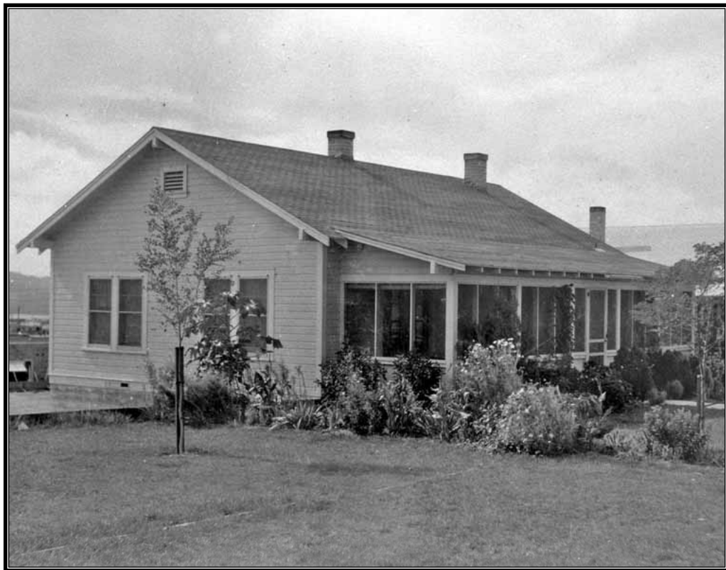
Figure 3.19 Five-room temporary frame residence shown in October 1933.
