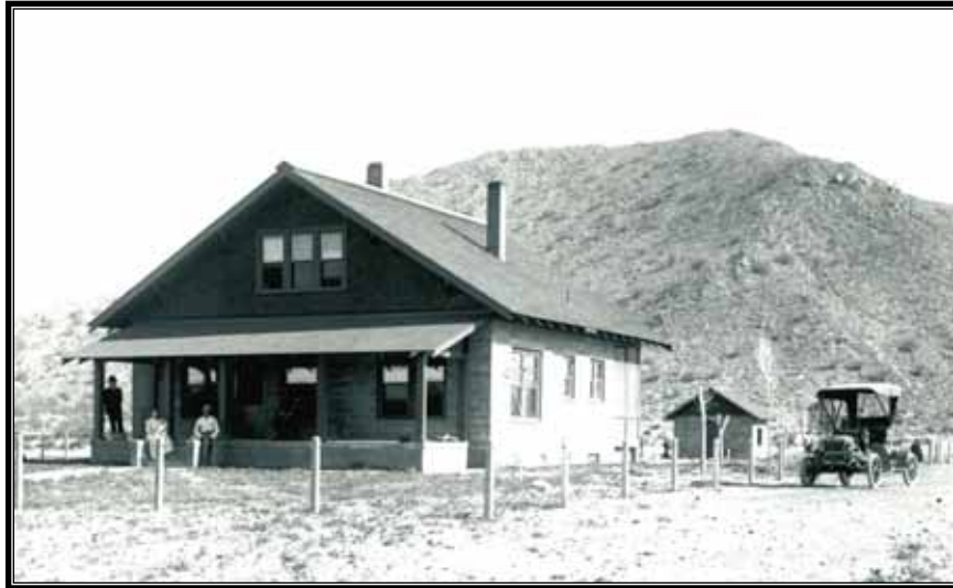
Figure 1.80 Salt River Project. Granite Reef dam tender's house, April 1910. This is the only known early Reclamation example of concrete block building construction. The house still stands.
