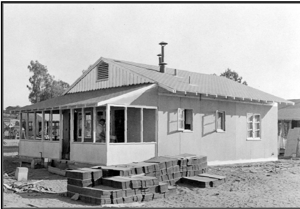
Figure 3.50 Nearly completed four-room, single-family residence at Friant Camp in October 1937.
