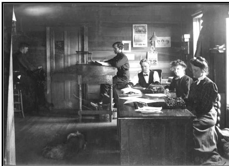
Figure 1.81 Uncompahgre Project. Temporary office building at Lujane, Colorado, 1907. Unpainted boards cover walls and ceiling.
