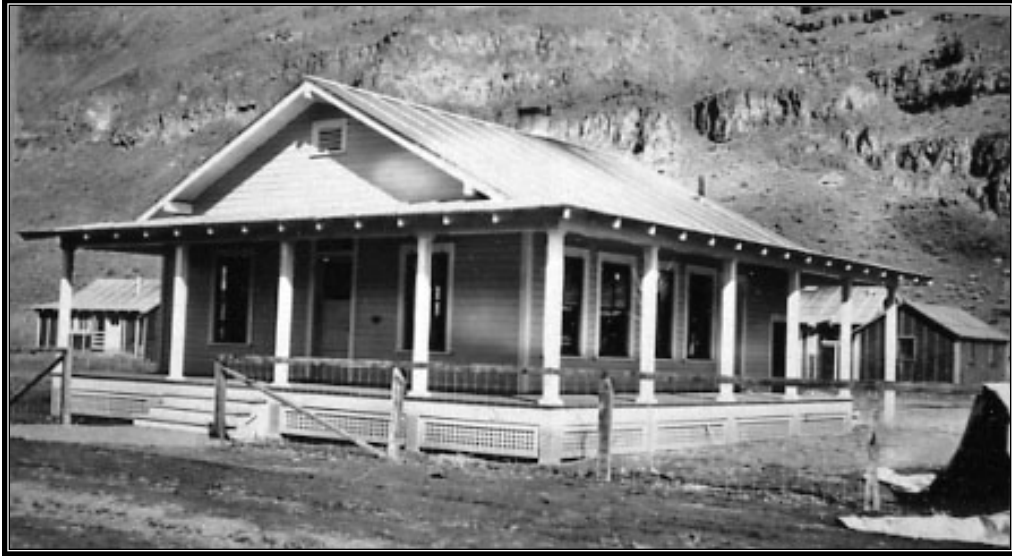
Figure 2.19 Owyhee Project. Office at Owyhee Dam site, 1928. (Source: Fred Quivik, Owyhee Dam, Historic American Engineering Record No. OR-17)
