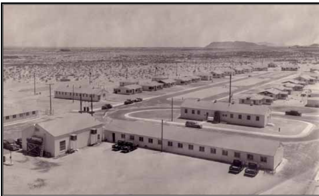
Figure 4.31 New Wellton Camp with residences laid out in a horseshoe plan around a center drive with parkways. Storage buildings in foreground.
