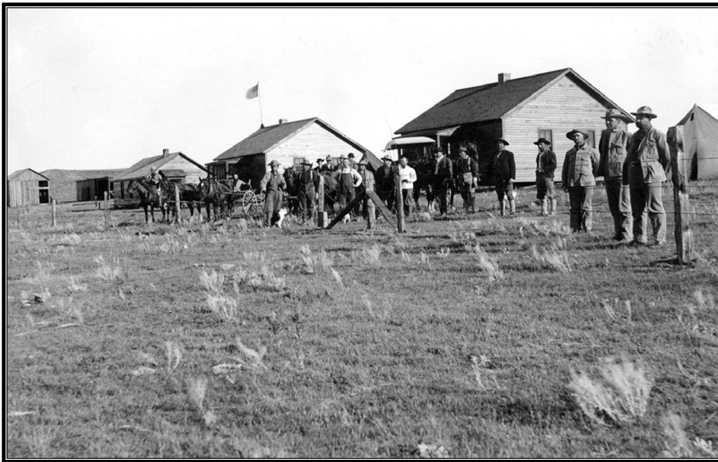
Figure 1.5 Belle Fourche Project, South Dakota. Owl Creek camp, August 1905. The simple frame buildings are arranged in an orderly fashion. Note the tent to the far right.
