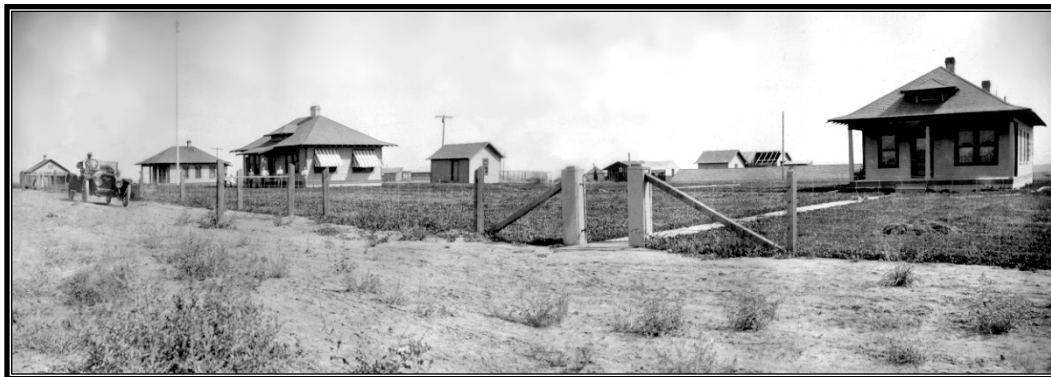
Figure 1.33 Yakima Project. Newly established headquarters for Tieton Unit on Naches Ridge, August 1911. The permanent hipped roof cottages with flared eaves, dormers, and simple columned porches are a more elaborate version of Reclamation's plain hipped box cottages. (Source: Upper Columbia Area Office, Bureau of Reclamation)
