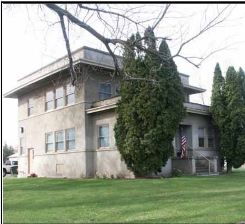
Figure 1.76 The Umatilla Project office has been occupied by the Hermiston Irrigation District since 1926. The building is still owned by Reclamation. (Source: Mark DeLeon, Bureau of Reclamation)
