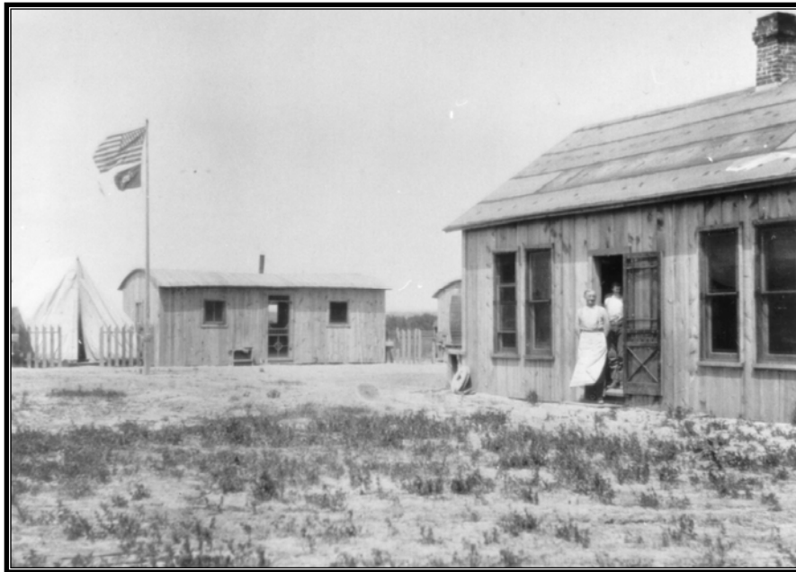
Figure 1.15 Belle Fourche Project. Temporary quarters for engineers, June 1905. Car-roof building with vertical board siding is at rear.
