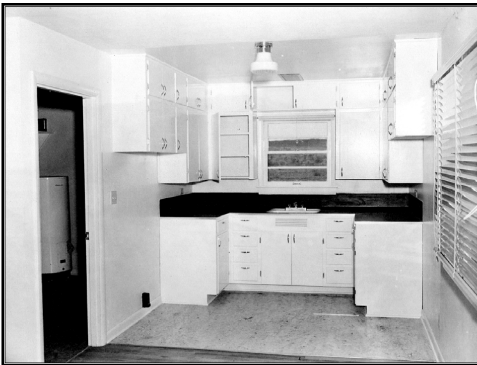
Figure 4.10 View of kitchen in ditchrider's house on Columbia Basin Project, August 12, 1951. Cupboards were prefabricated.
