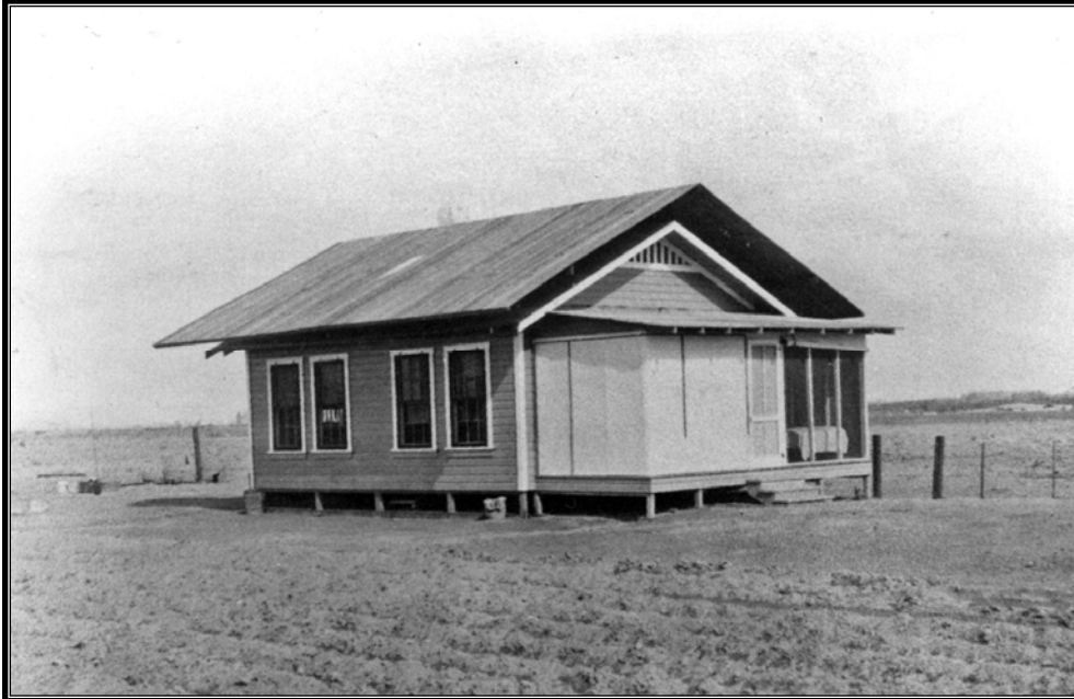
Figure 2.16 Yuma Project. Permanent ditchrider's house on the Valley Division of the Yuma Project, 1921. Construction history is unknown, although it likely dates from mid- to late teens.
