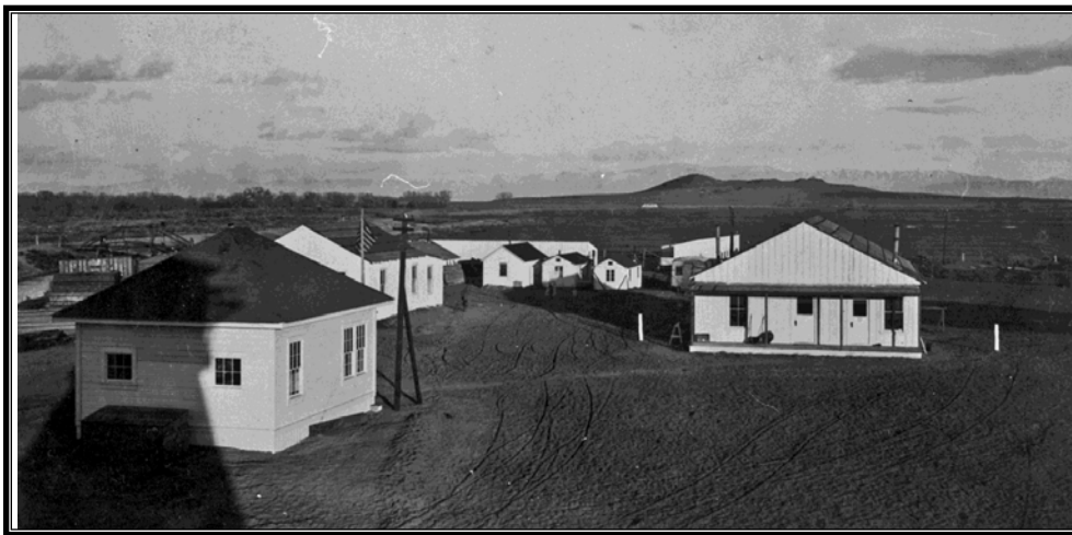
Figure 1.13 Newlands Project, Nevada. Headquarters in Fallon, 1907. This original project headquarters complex consisted of a variety of temporary buildings. The office is the hipped roof building at left. Permanent headquarters were established at a new site in Fallon in 1910.
