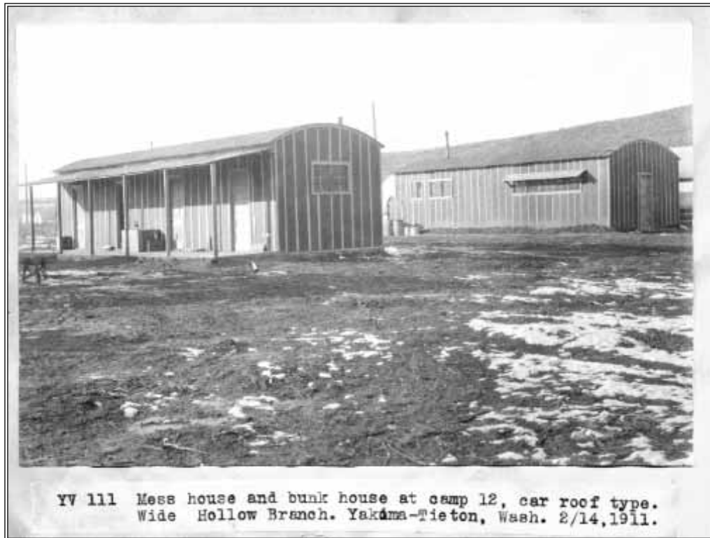
Figure 1.17 Yakima Project. Car-roof buildings covered with tar paper, February 1911. (Source: Upper Columbia Area Office, Bureau of Reclamation)
