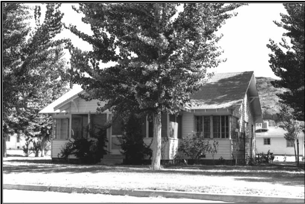
Figure 4.29 Parker Dam Camp. House number 55, built in 1948, evokes the earlier Bungalow form. Photo date unknown.
