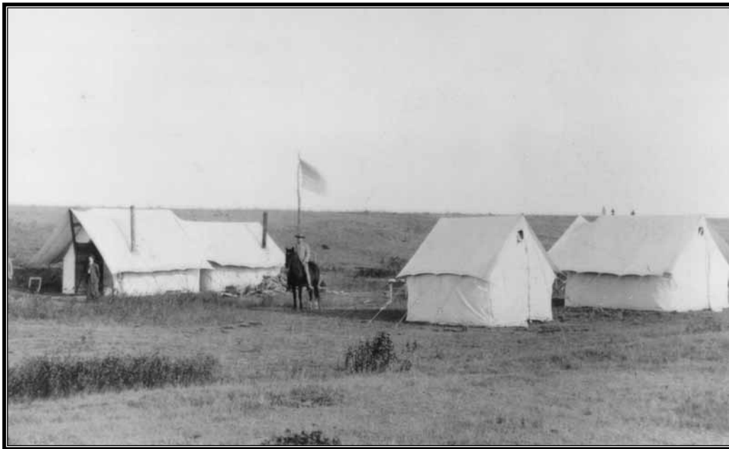
Figure 1.1 Lower Yellowstone Project, Montana. Headquarters at Newlon, October 11, 1904. Temporary wooden buildings replaced tents in the summer of 1906.
