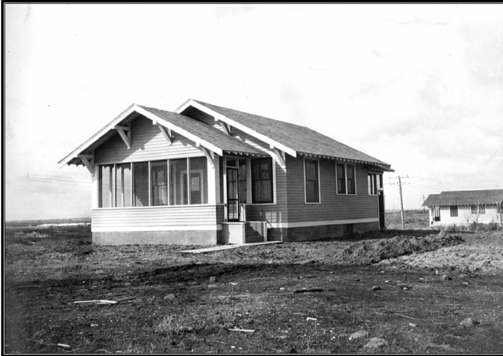
Figure 1.88 Minidoka Project. Three-room permanent Bungalow cottage built at Minidoka Dam camp in 1914. Three identical cottages were built at a total cost of $5,298.
