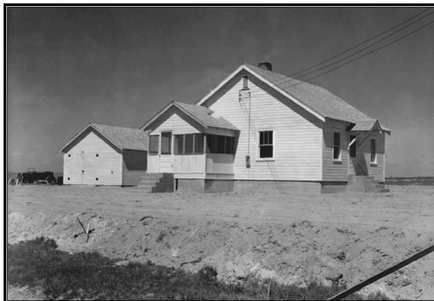
Figure 3.63 Boise Project. Ditchrider's house on the Payette Division, 1941.
