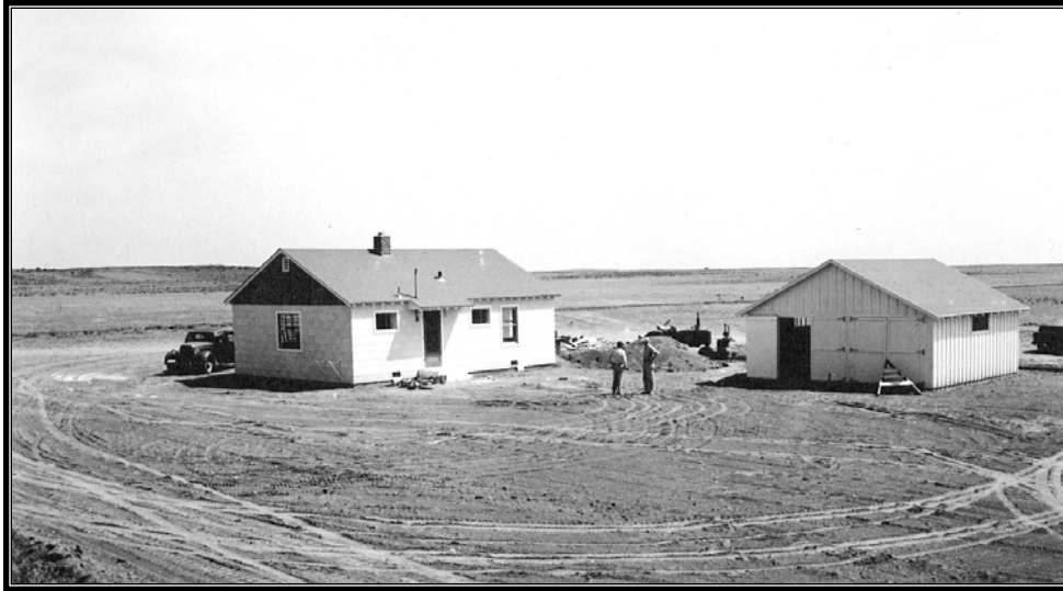
Figure 4.9 New ditchrider's house near Gloyd, Washington. Photo taken June 6, 1951.
