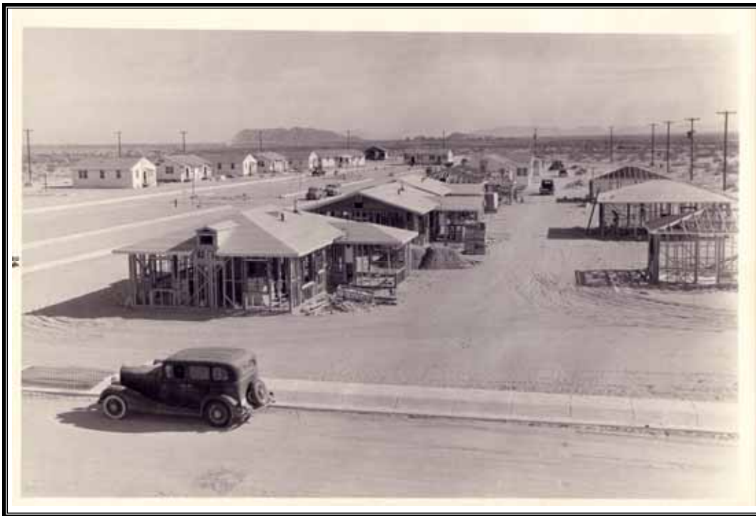
Figure 4.30 Gila Project. Residences at Wellton Camp under construction.
