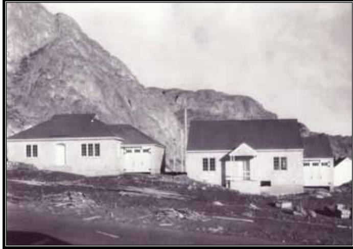
Figure 3.24 First permanent residences at Coulee Dam under construction in 1934. On the left is a four-room house with a gable-on-hip roof (drawing number 222-D-396). On the right is either a three- or four-room house with side-gabled roof. Both house types in this photograph would be built on other Reclamation projects.
