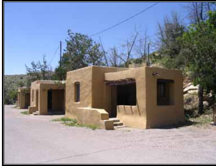
Figure 3.76 CCC tourist cabins at Elephant Butte Reservoir, 2007. (Source: Christine Pfaff, Bureau of Reclamation)
