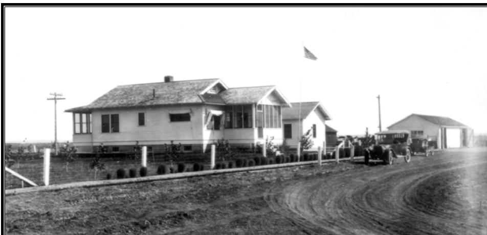
Figure 2.8 Milk River Project. A variation on the 1918 standard four-room cottage design was used for an office and lodging house in Saco, Montana. Photo taken in 1922.
