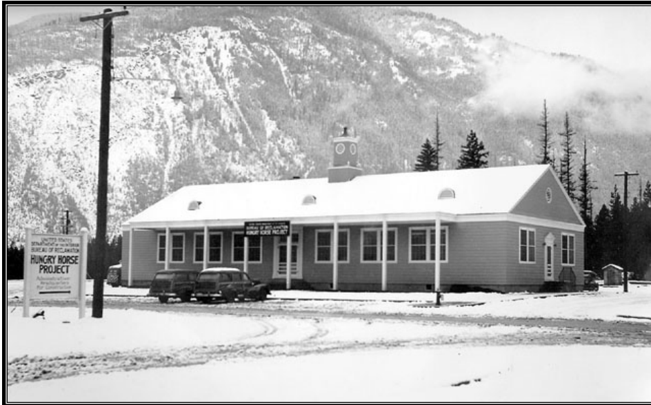
Figure 4.15 Hungry Horse Project. Administration building repeats design of offices in Estes Park, Colorado, and Toyon, California. Photo taken on November 14, 1947.
