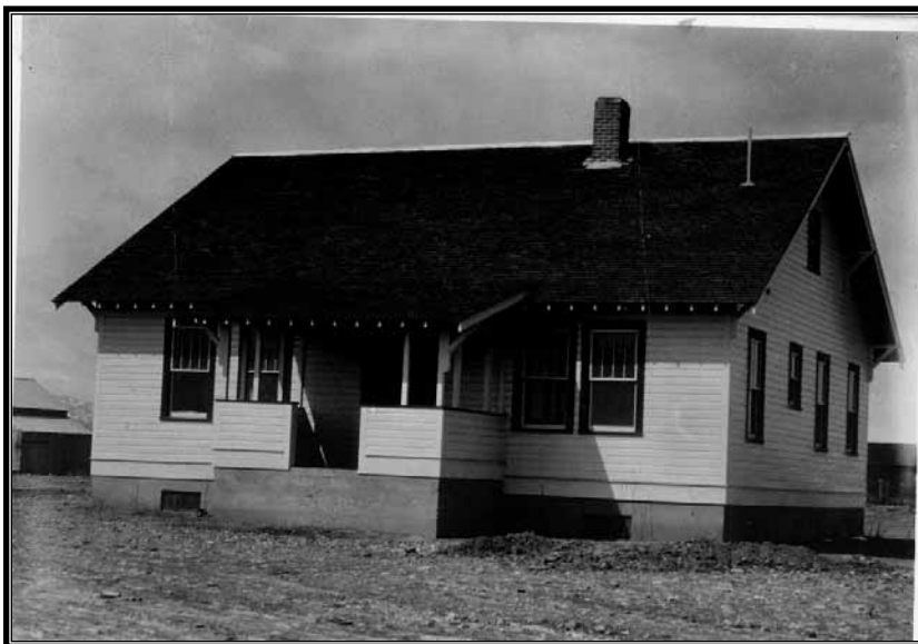
Figure 3.3 Shoshone Project. The 1931 Willwood Division office building designed in the Denver office bears similarities to the 1918 standard three-room cottage plan. The 1918 standard drawing for wall and mill details (40-C-77) was specified for the interior. Photo taken on April 30, 1932. (Source: Shoshone Irrigation District)
