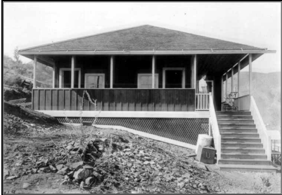
Figure 1.48 Salt River Project. Mr. Smith's cottage, November 1905. The moderately pitched hipped roof incorporates a wraparound porch. The cottage probably was occupied by Chester Smith, Reclamation construction engineer, and his family.
