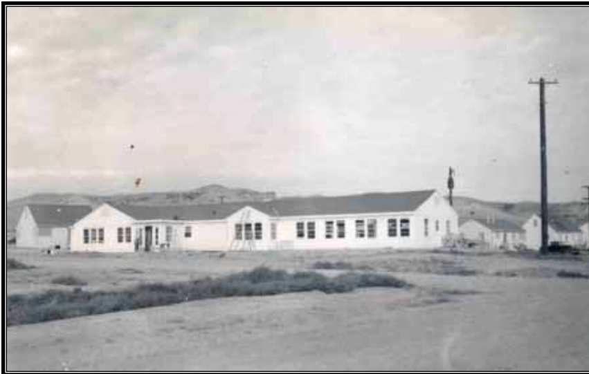
Figure 4.20 Tiber Dam government camp. Reclamation construction field office. Photo taken September 12, 1952.
