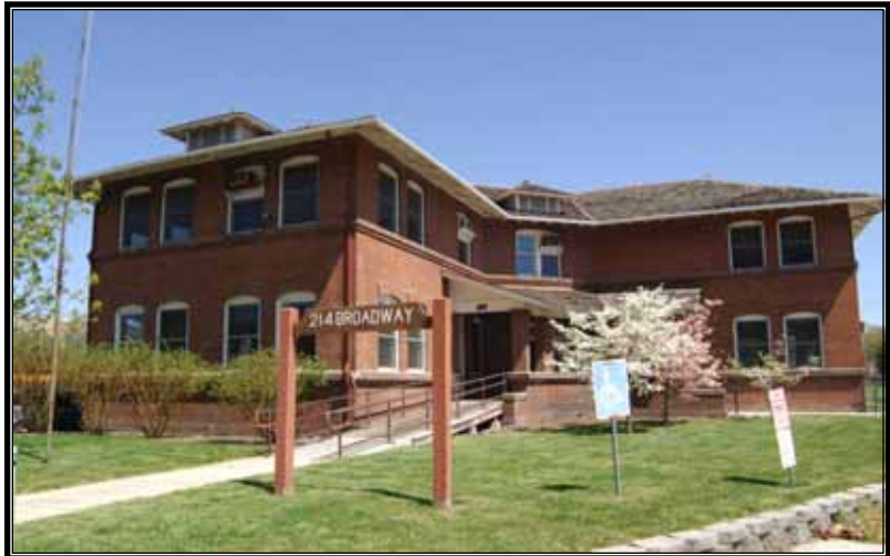
Figure 1.73 Boise Project office in 2007. In 2006, Reclamation transferred the building to the Idaho Historical Society. (Source: David Walsh, Bureau of Reclamation)
