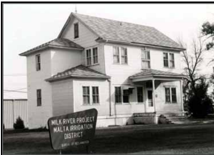
Figure 1.57 Milk River Project. Headquarters building in Malta, Montana. Just visible to the left side is a two-story concrete vault original to the building. Deviations in construction from the original blueprints were numerous and included Doric columns rather than turned porch posts, a reference to the Colonial Revival style.
