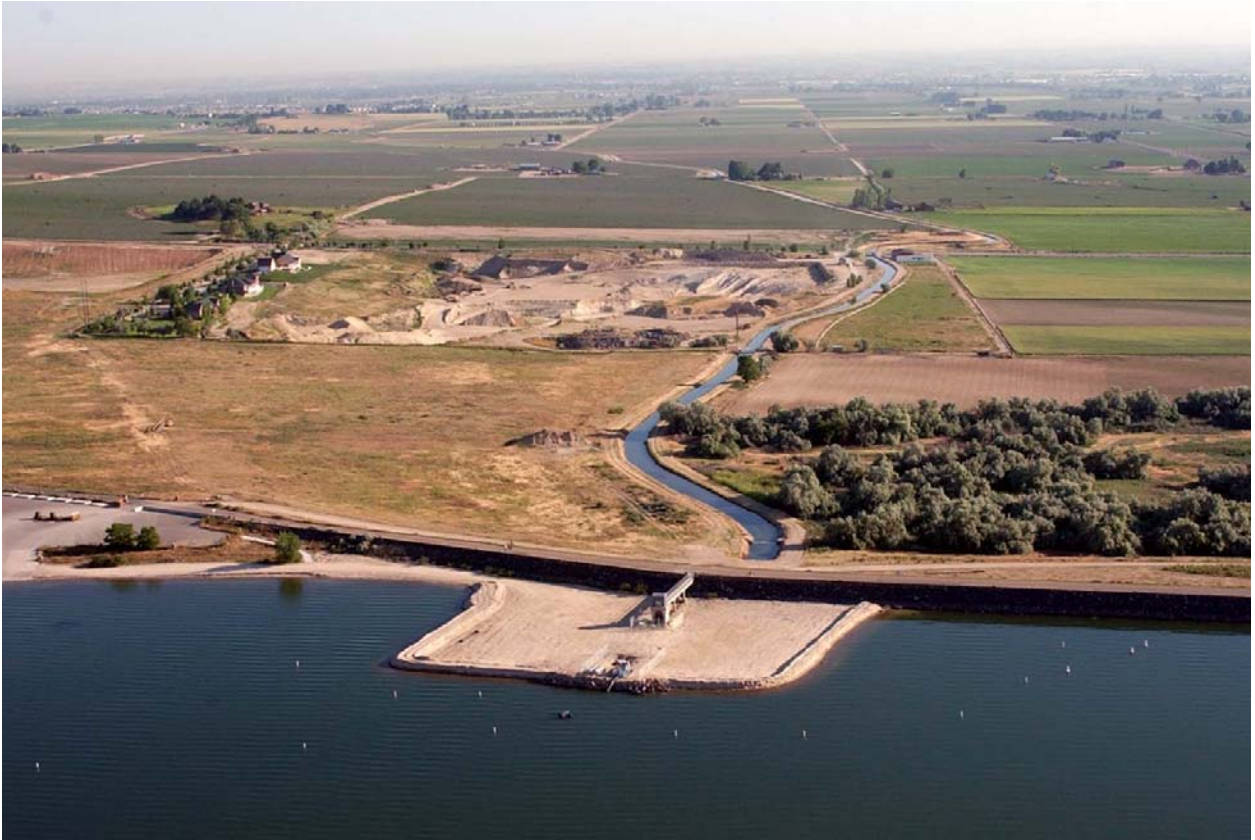
Figure 2 - View to the north showing the earthen emergency berm surrounding the Caldwell Canal gate control tower. Pumps are visible in the foreground. Area proposed for temporary stockpile of excavated material is to the left of the canal.
