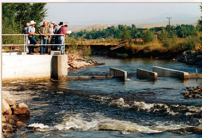
New irrigation diversion, Central ID
