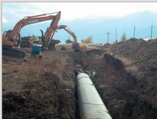
Medford Irrigation District - installation of pipeline.
