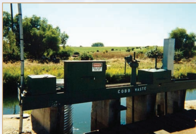
Old headgate structure after efficiency improvements
