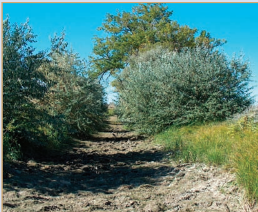
Paradise Valley Irrigation District Hillside ditch lateral to be replaced by buried pipe.
