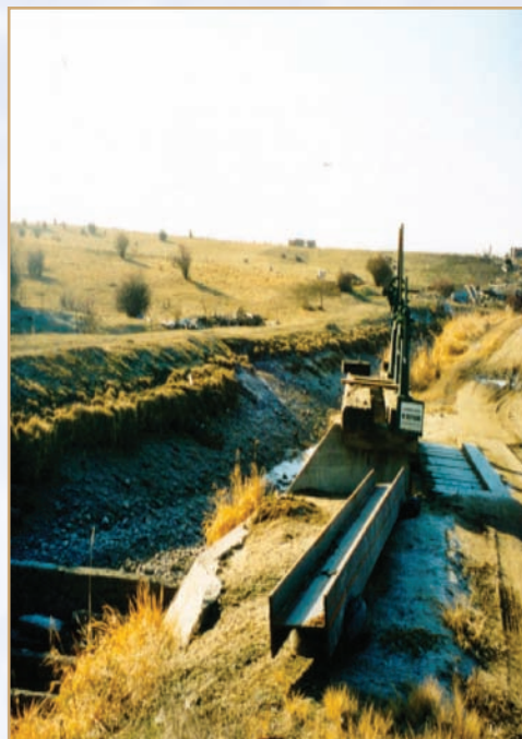
Old headgate structure before improvements
