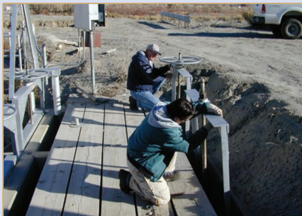
Emery Water Conservancy District - installation of automation equipment.
