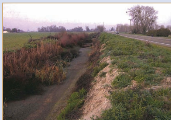
Stevinson Water District - dirt canal to be replaced by pipeline.
