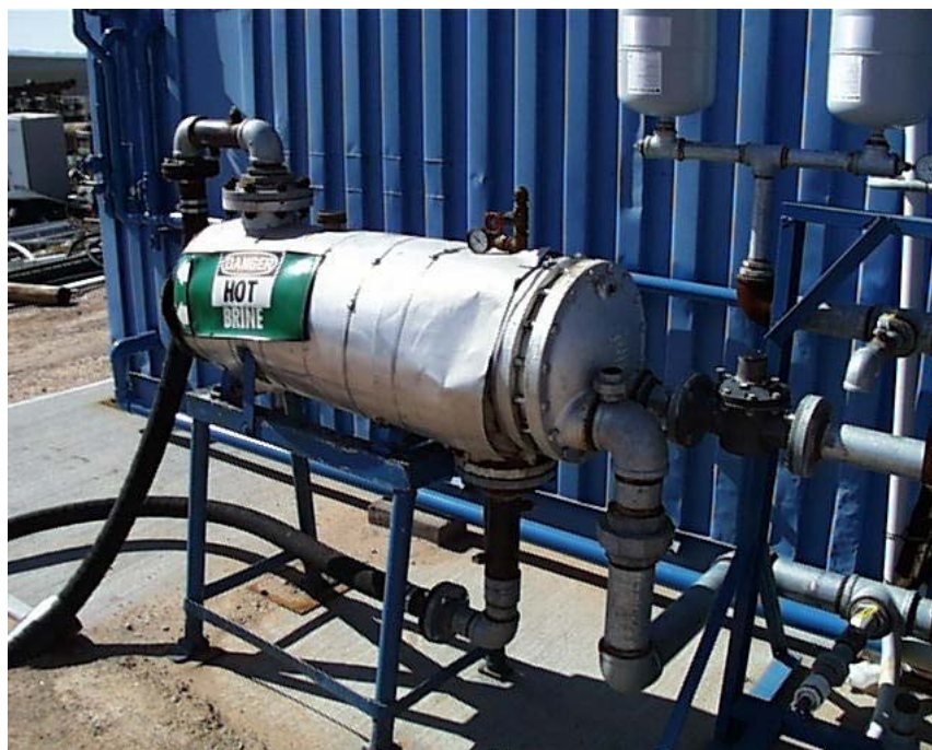
Figure 13.—Intermediate heat exchanger.
