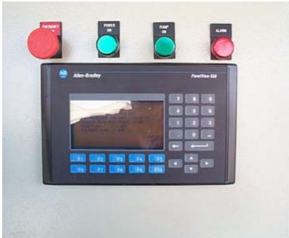
Figure 5.1.—Memcor PLC Screen
