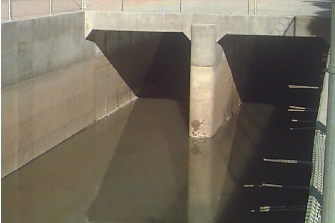
Figure 4.1.—Franklin Canal located adjacent to El Paso’s Canal Street Plant
