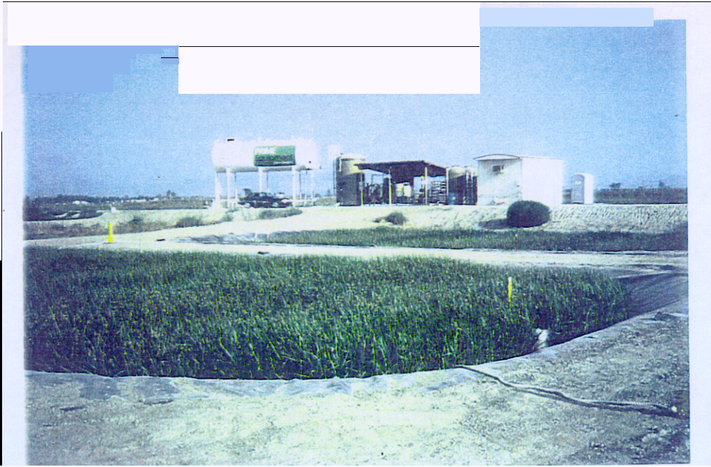
Figure 2.6.—RO pilot plant with saline wetlands shown in the foreground.
