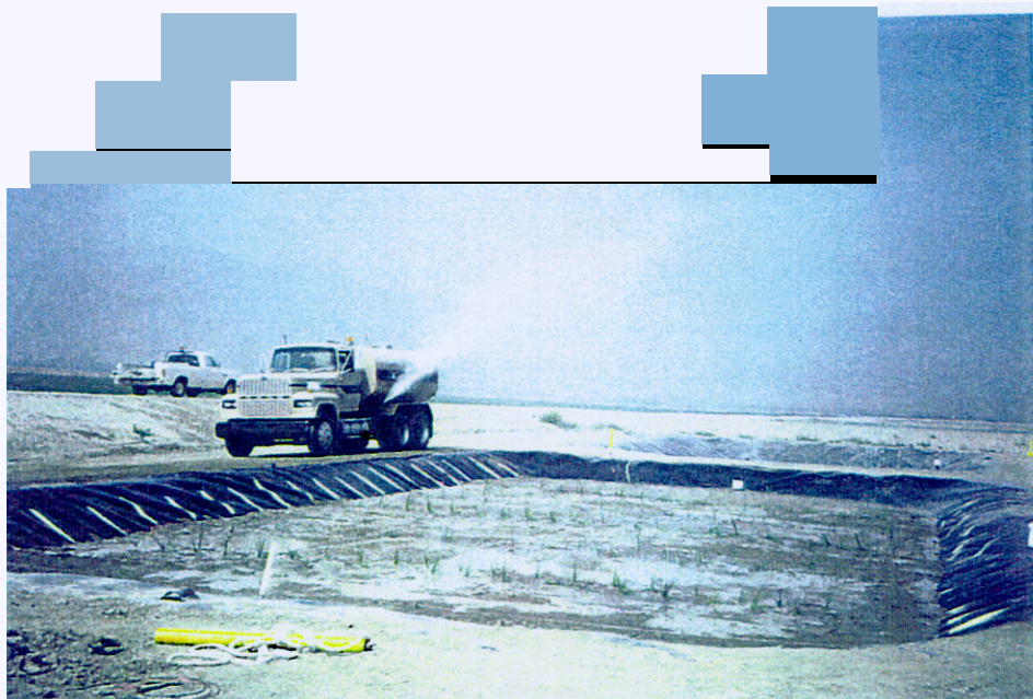
Figure 5.6.—Potable water being applied to the newly planted saline wetlands to promote plan establishment.
