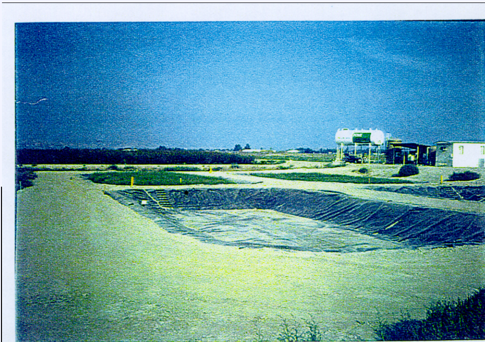
Figure 6.1 .-North evaporation pond with adjacent, upstream vegetated wetlands and RO unit in the background.
