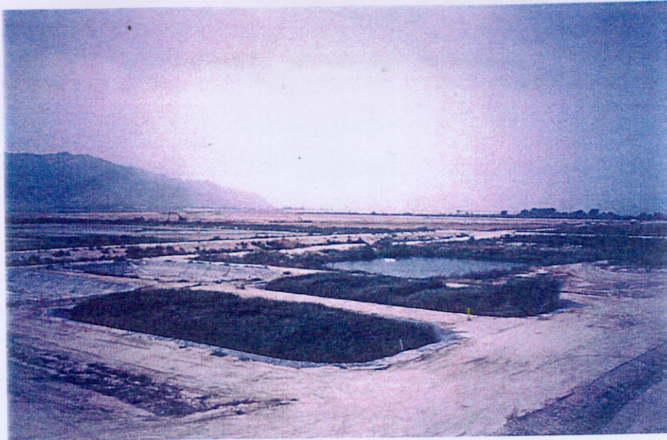
Figure 5.7.—View of both vegetated wetlands during May 1994 showing very lush, vigorous, and healthy plant growth (south cell had not received RO reject since February 9, 1994).
