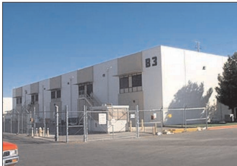
Figure 1.3.1-4: Exterior view of building B3.
