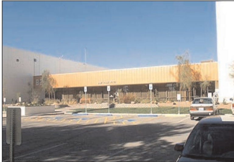
Figure 1.3.1-3: Exterior view of building B2.
