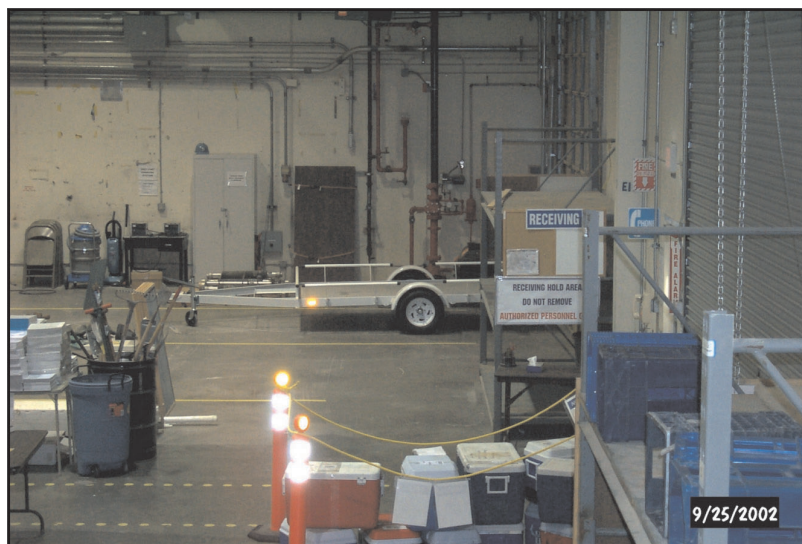
Figure 2.2.2-3: IT/SHAW shipping/receiving area in the B1 high bay.
