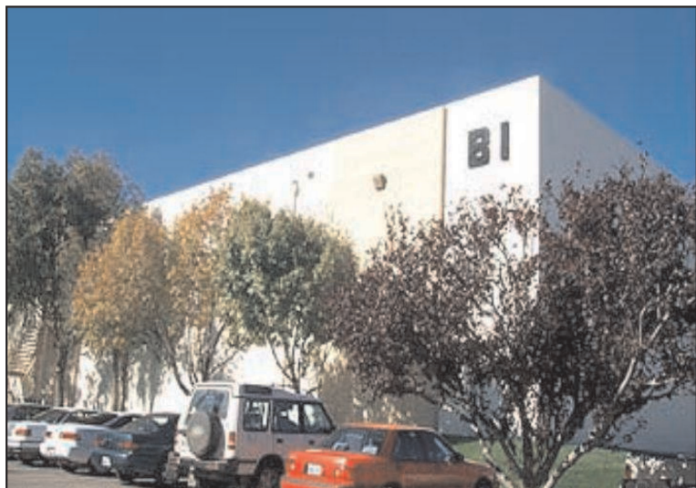
Figure 1.3.1-2: Exterior view of building B1.
