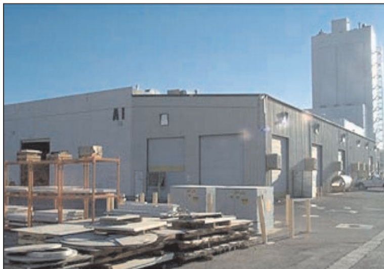
Figure 1.3.1-5: Exterior view of building A1.
