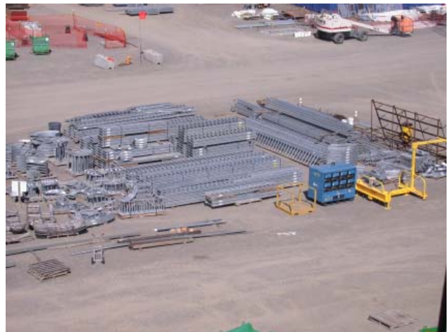
A properly maintained lay-down area
