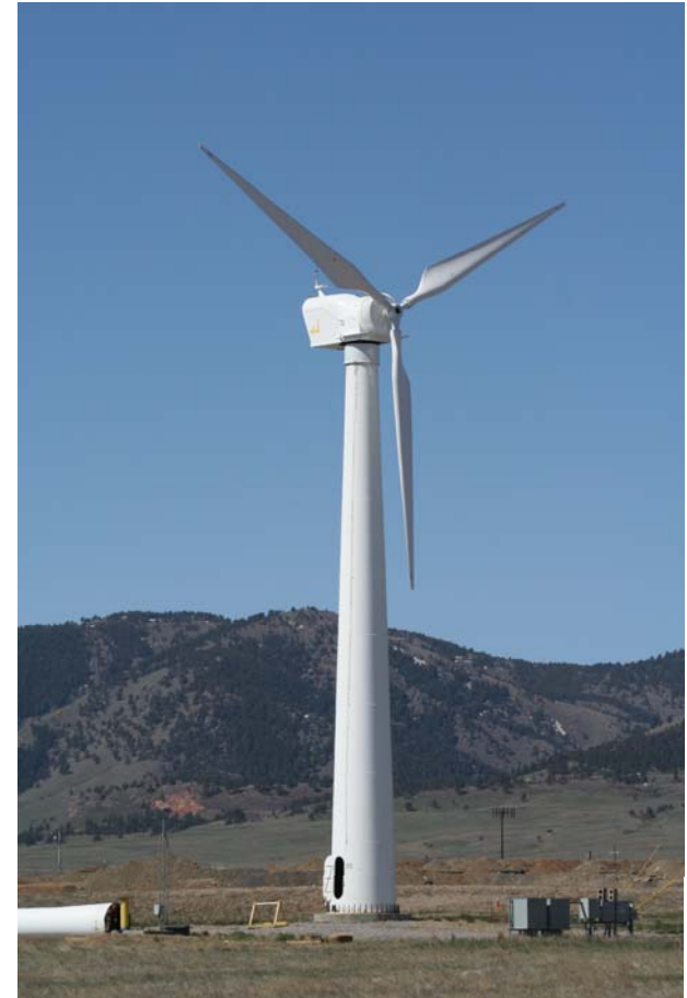
NW100B 100-kW wind turbine
