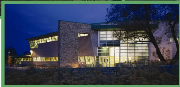
Center for Integrated Nanotechnologies Los Alamos National Laboratory & Sandia National Laboratory
